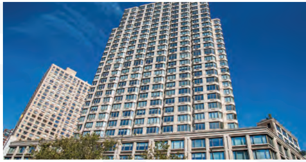
FIGURE 2: CarbonQuest installed their CCUS in a 377,000-sq-ft multi-family unit in Manhattan with a goal to reduce CO 2 emissions by 25% and provide a 5-year return on investment (ROI). Courtesy: CarbonQuest
