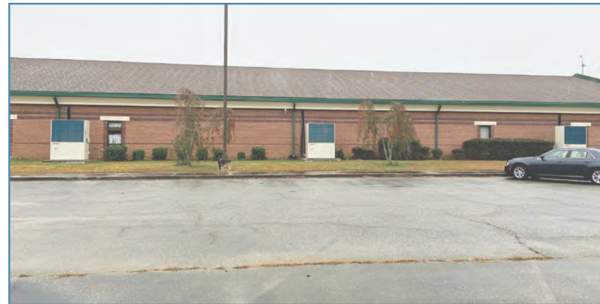
FIGURE 3: City of Dublin Natural Gas is the natural gas provider for the Dublin City Schools. The City’s financing program proved instrumental to the overall project success. Courtesy: Dublin City Schools and Clay Consulting
