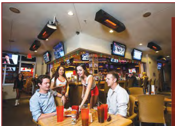
Dining areas that are open to the outdoors or have high ceilings can increase customer comfort by applying infrared tube heaters. Photo courtesy: Schwank USA.
