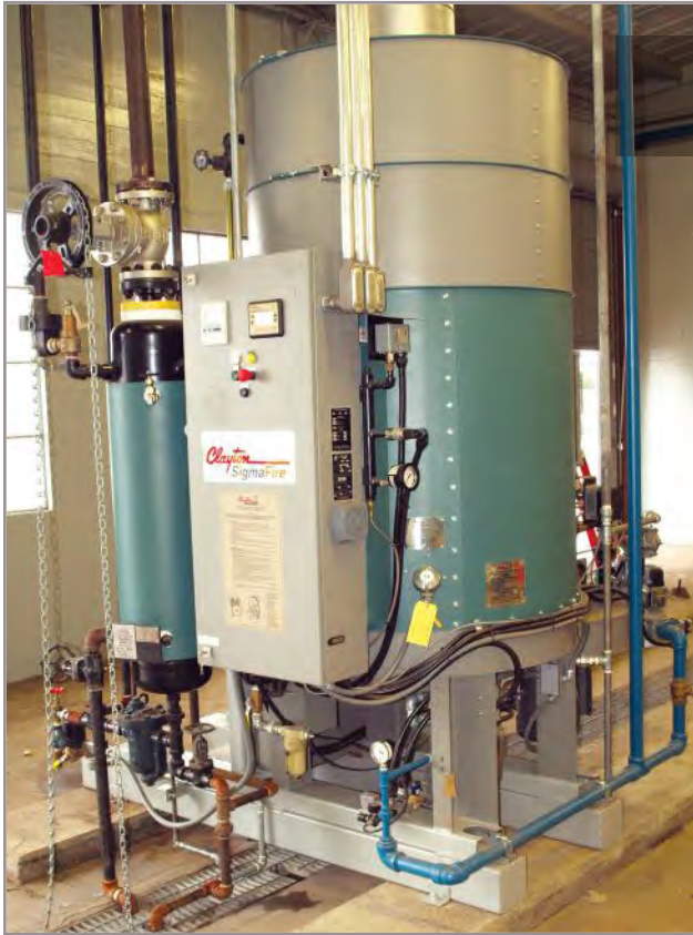
Vertical package boilers are especially attractive because of their minimal floor space requirement. Photo courtesy: Clayton Boilers.
