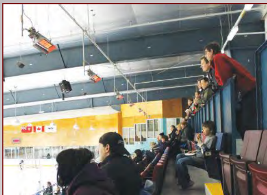
Hockey, football and other athletic venues benefit from overhead infrared heat. Tube heaters can be effective at heights up to 180 feet. Photo courtesy: Schwank USA.
