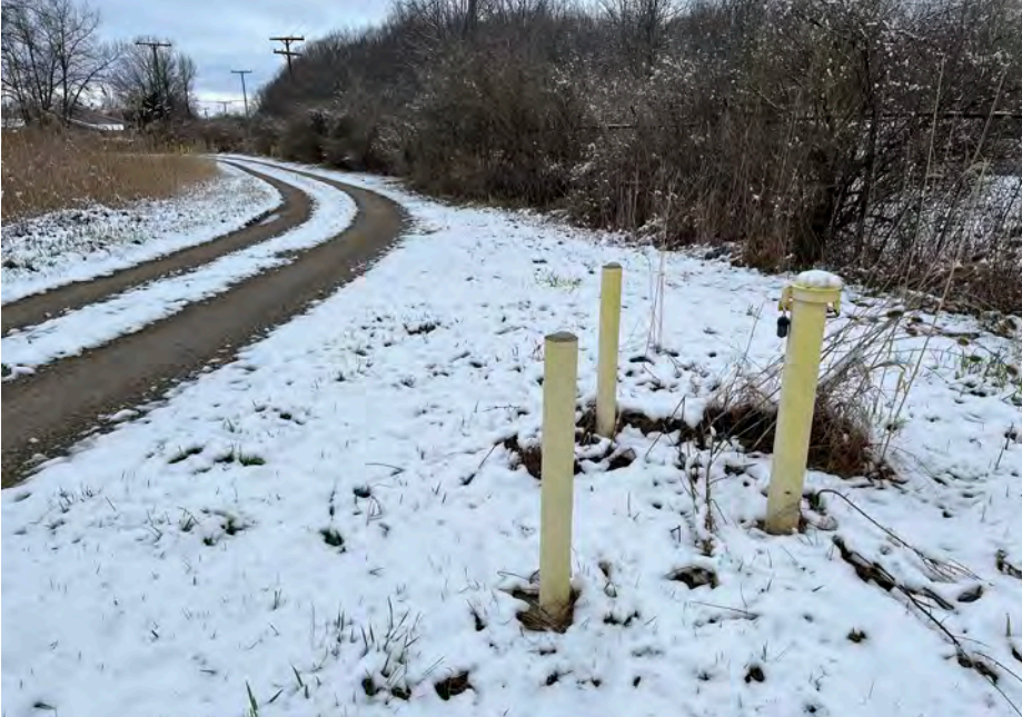
13. Monitoring Well and Perimeter Road Along Northeast Corner. Road in Good Condition and Well Locked.
