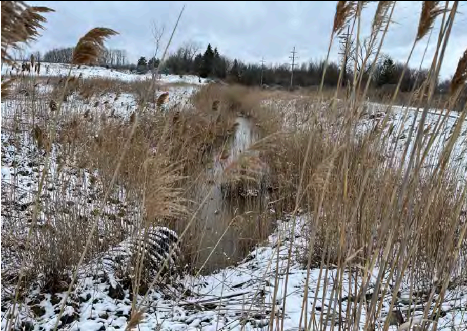
9. Flow from Culvert into Perimeter Ditch. Culvert and Ditch Remain Open.
