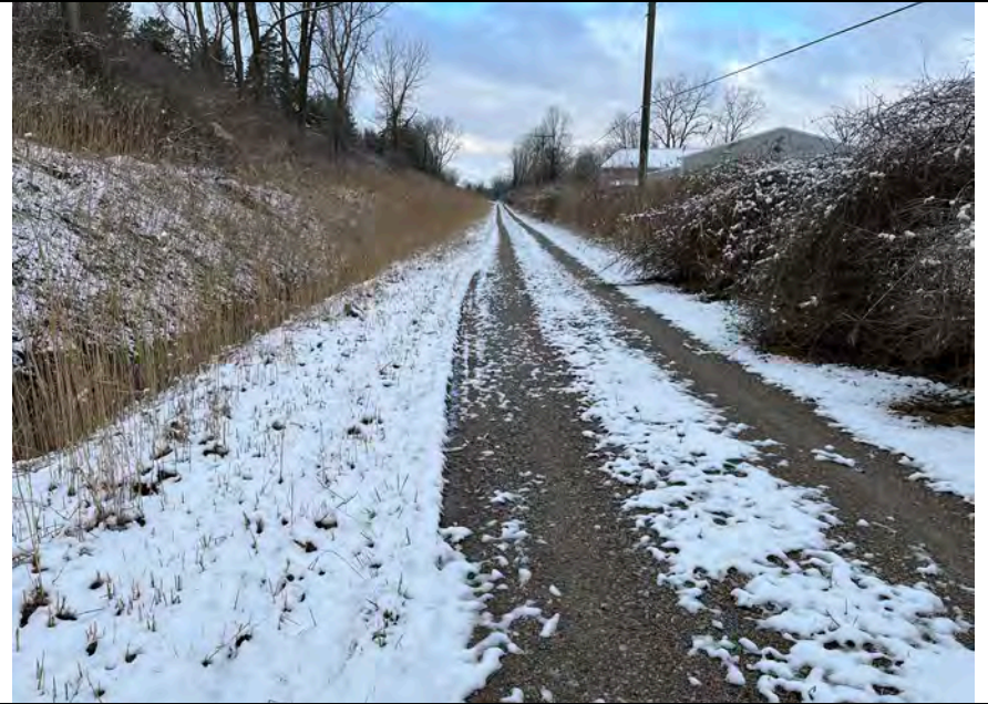
18. Ditch Alignment and Perimeter Road in Good Condition. Trees Along Outside Slope of Closed Landfill Areas at North End of Landfill.
