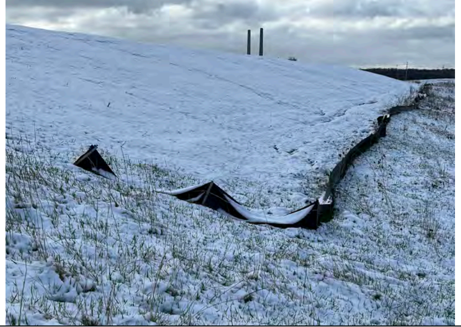
30. Western Side of Area G2 Graded and Seeded. Some Minor Slope Runoff Erosion Shown and Should be Observed and Inspected As Vegetation Grows.
