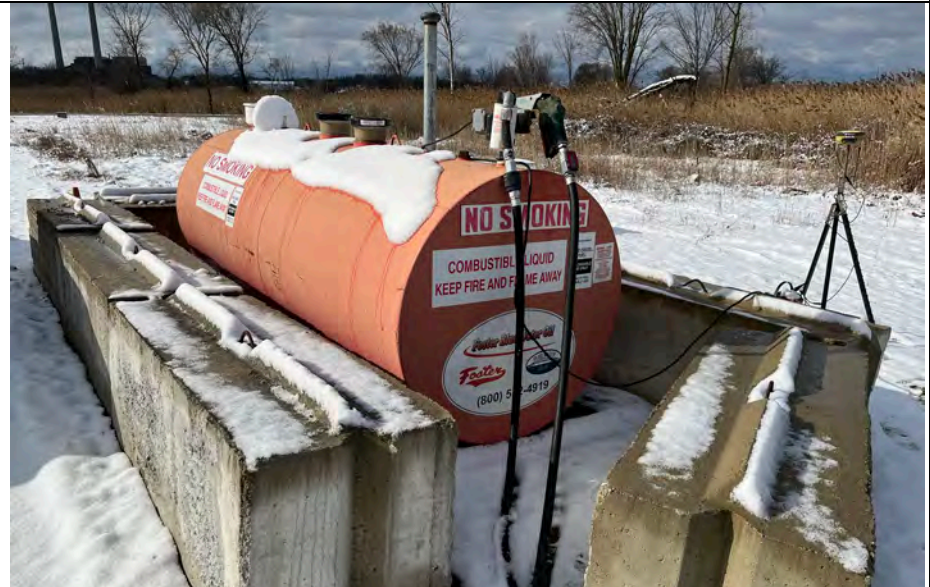
8. Single AST at Contractor Onsite Yard/Office. No Leakage Observed.
