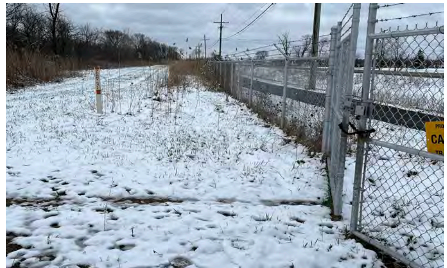
28. West Side Access Fence, Locked and Signage Posted. Perimeter Slurry Wall Marker Shown.
