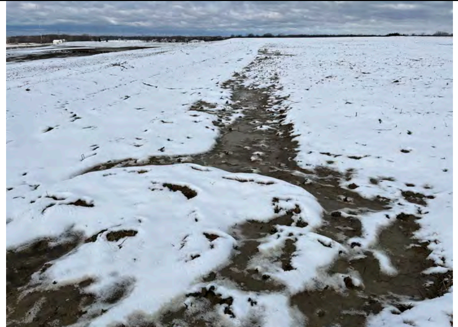
38. Surface Drainage Swale Top Area G2 Phase 1 with Slope into Phase 2. Some Rutting but Repair/Re-seeding Completed in Spring 2022, per DTE.
