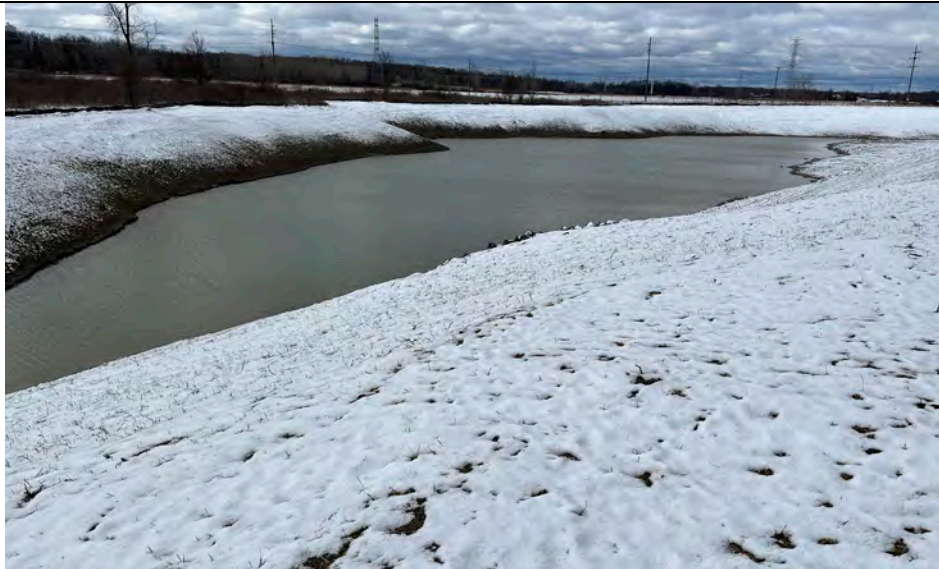
43. Runoff Pond Constructed Southeast of Active Area G2 Phase 2.
