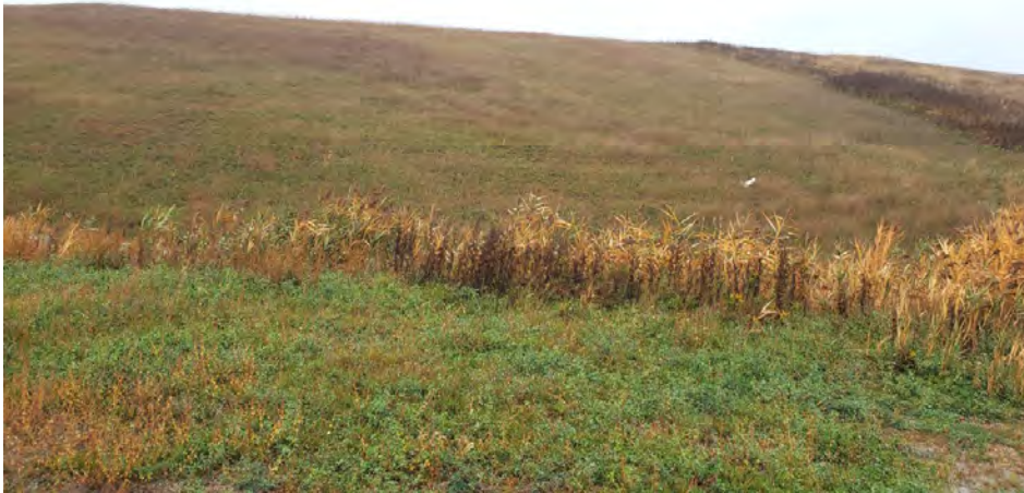
41. DTE Photo of Area G2 Phase 1 Slope after Seeding Growth and Typical of Slope and Cover Seeding and Spring Re-Seeding.
