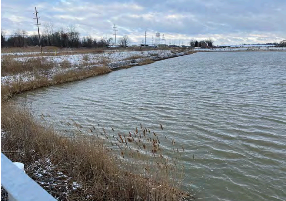
1. Storm Water Detention Basin (SWDB), S & W Sides. Slopes are Protected with Stone. No Visible Slope Erosion on All Sides. Same for N & E Sides.
