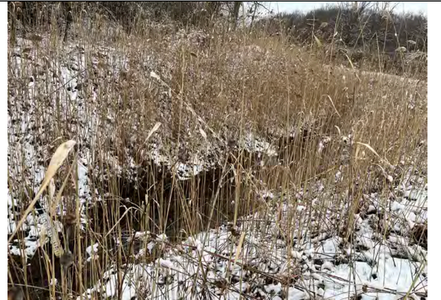
12. Perimeter Ditch at Corner with Vegetation but Still Open.
