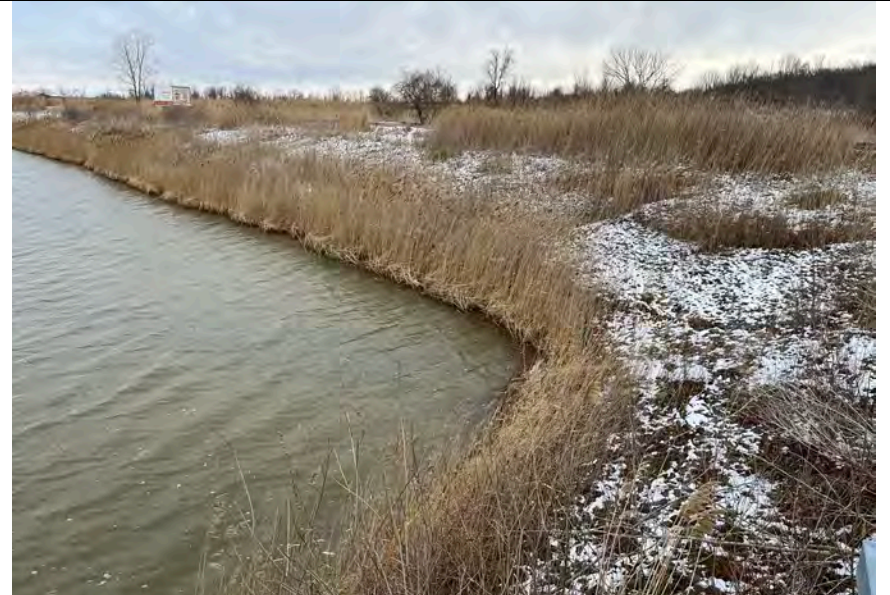
4. Looking at NE Corner of SWDB. Slope Protected from Erosion with Stone. Staff Gauge SG-13 in Middle of Photo at or Just Above the Water.
