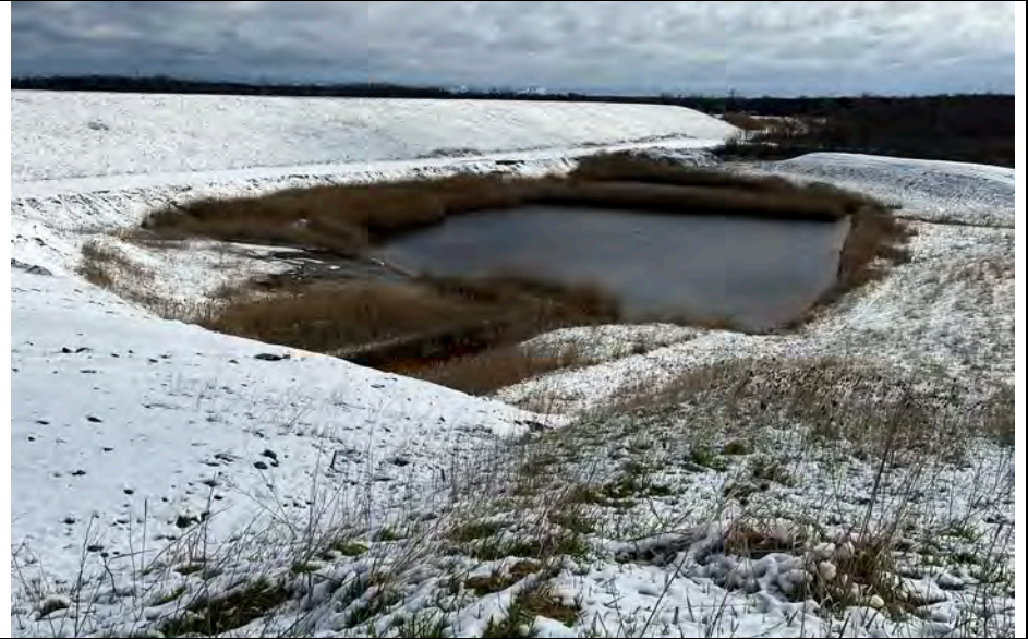
36. Central Runoff Holding Ponds. No Blockage Observed and Ditch Vegetation Appeared Satisfactory Although Not Walked Due to Slip, Trip & Fall Safety.
