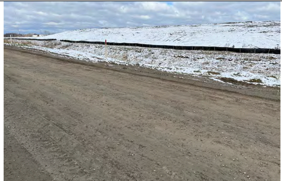
47. Haul Road in Excellent Condition and Internal Drainage Ditch Outside of Landfill Silt Fence. Silt Fence in General Satisfactory Condition.
