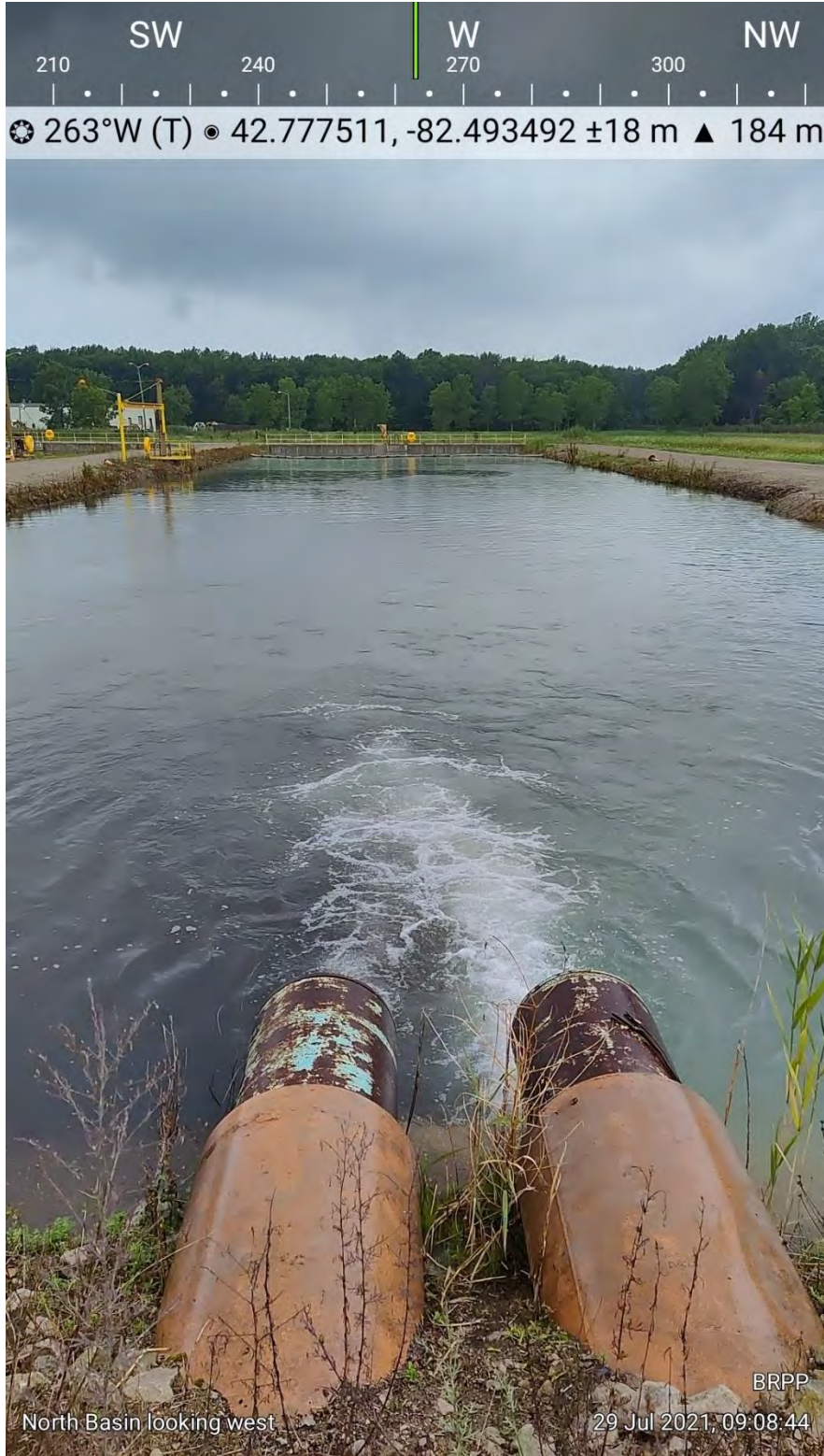
Photograph 1: North Basin Looking West from the East End of the Basin
