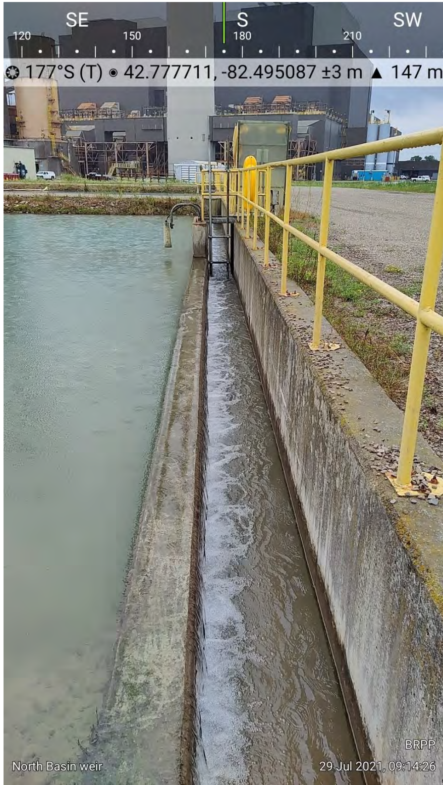
Photograph 4: North basin Weir Looking South from Northwest Corner of Basin
