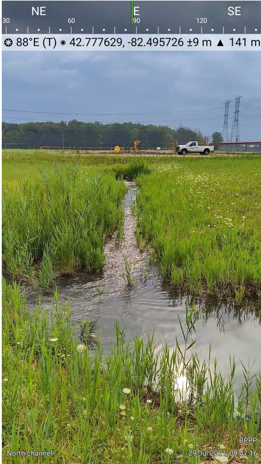
Photograph 7: North Discharge Channel Joining Flow From South Discharge Channel Looking East from West of the North Basin
