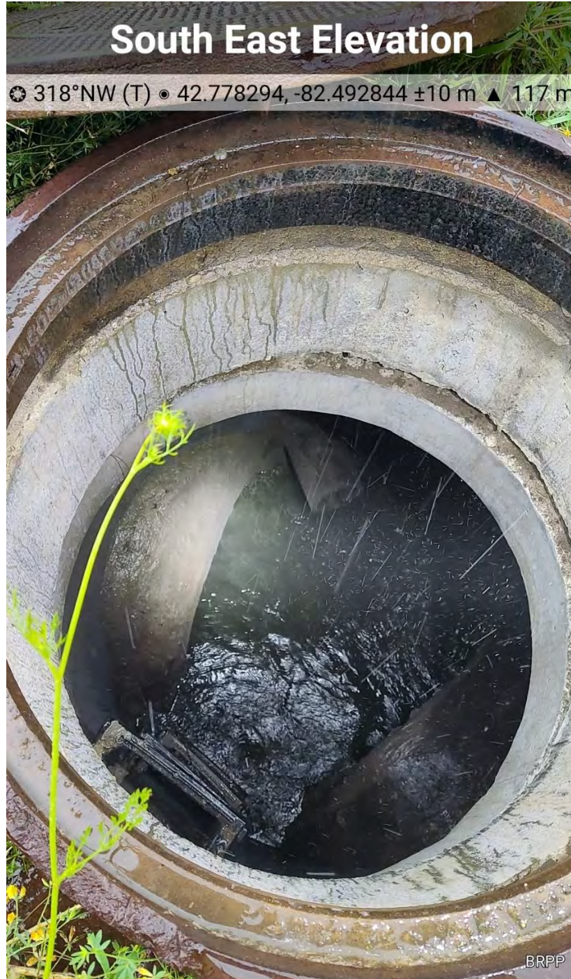
Photograph 10: MH-1 Junction of Flows from Basins and RRLF
