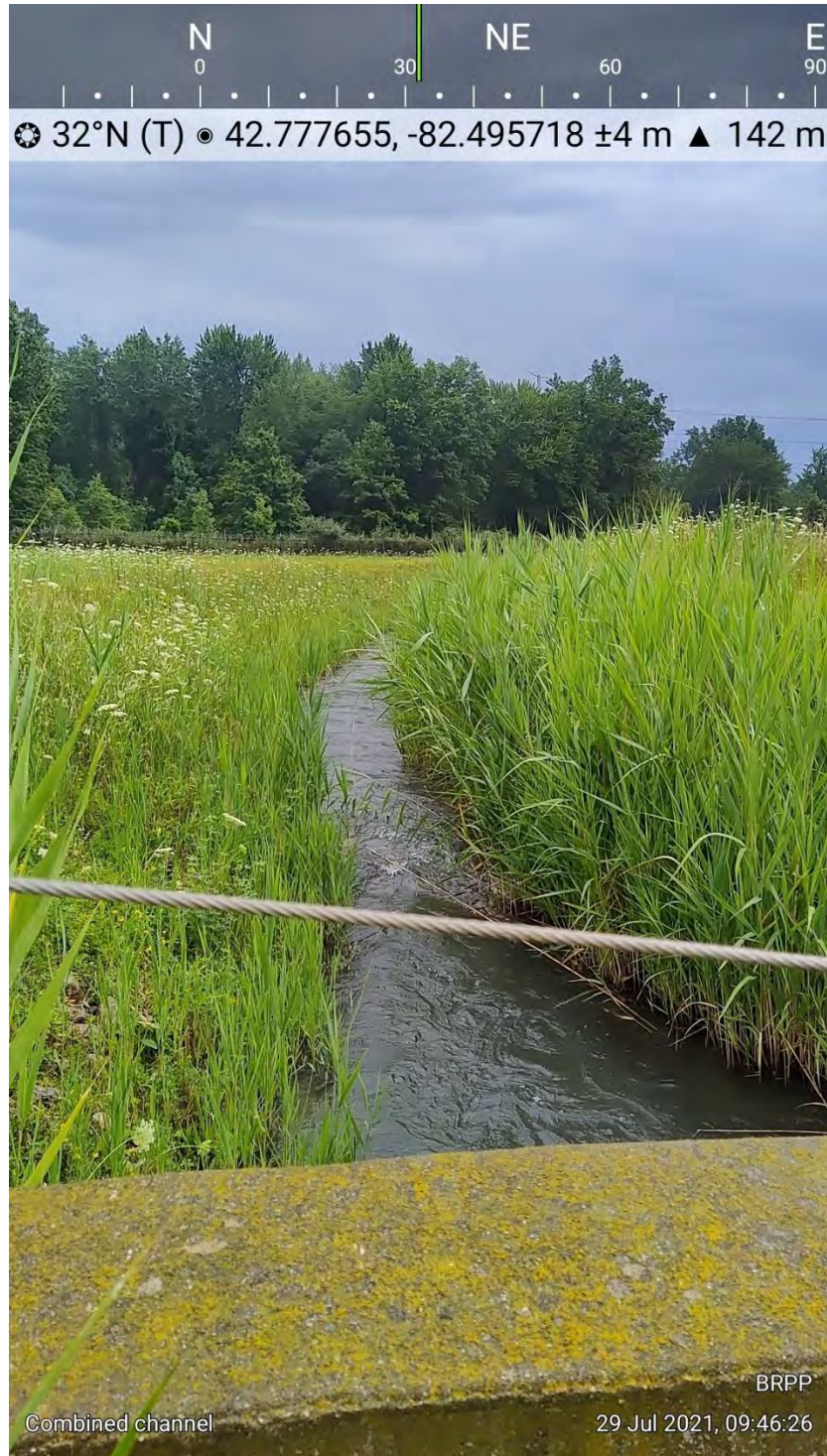
Photograph 8: Combined Discharge Channel Looking Northeast from the Knife Gate
