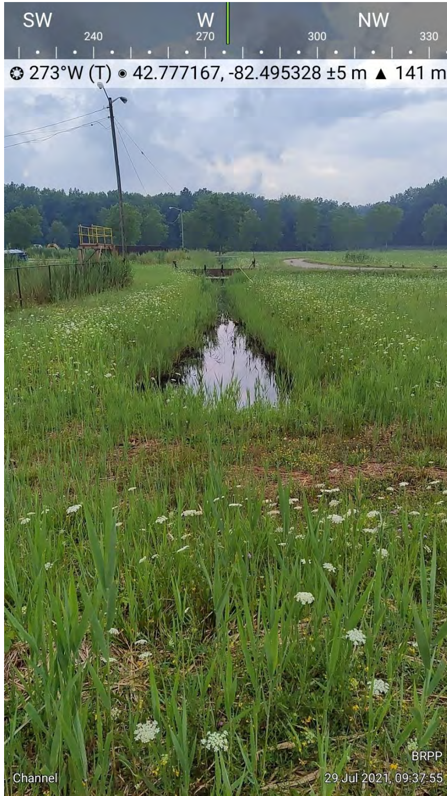
Photograph 5: South Discharge Channel Looking West from West End of South Basin
