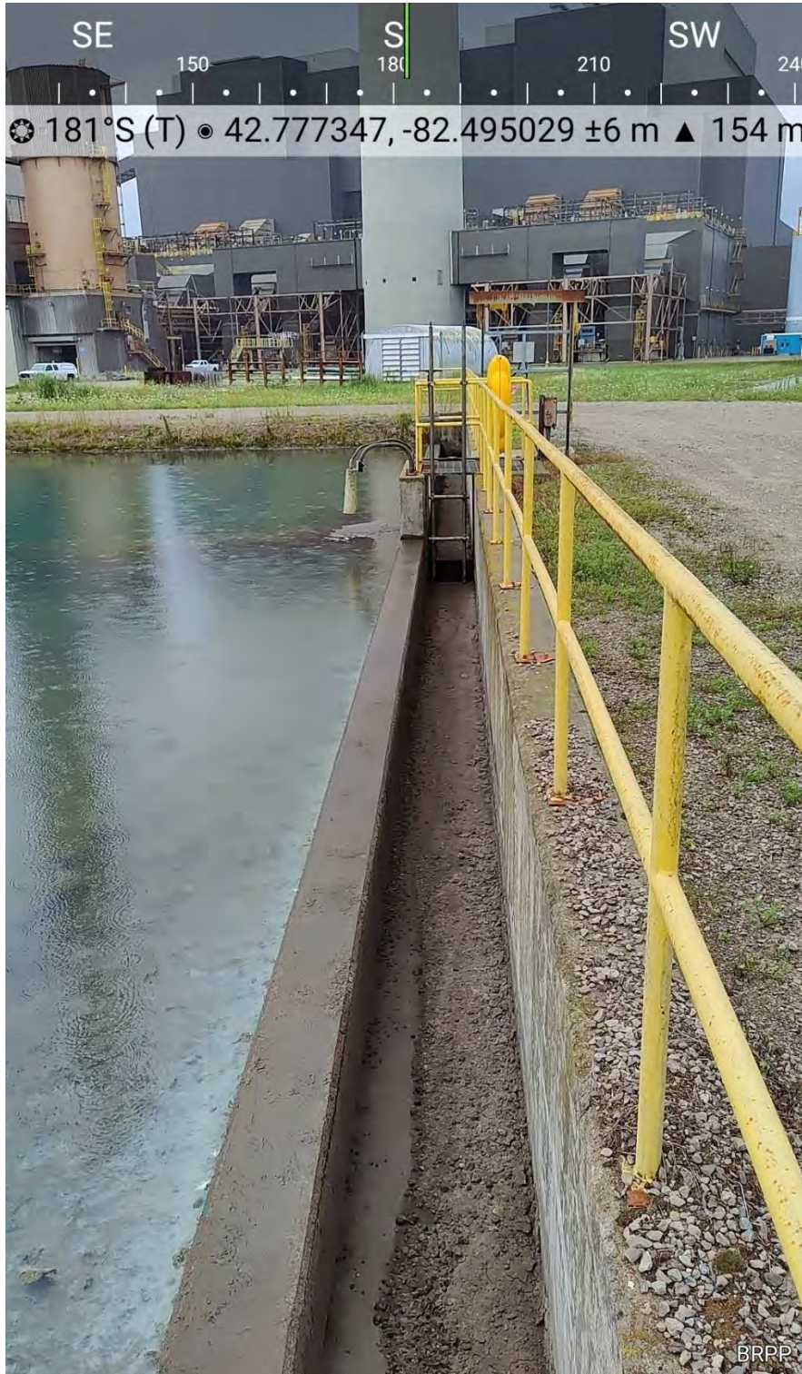
Photograph 3: South Basin Weir Looking South from Northwest Corner of South Basin
