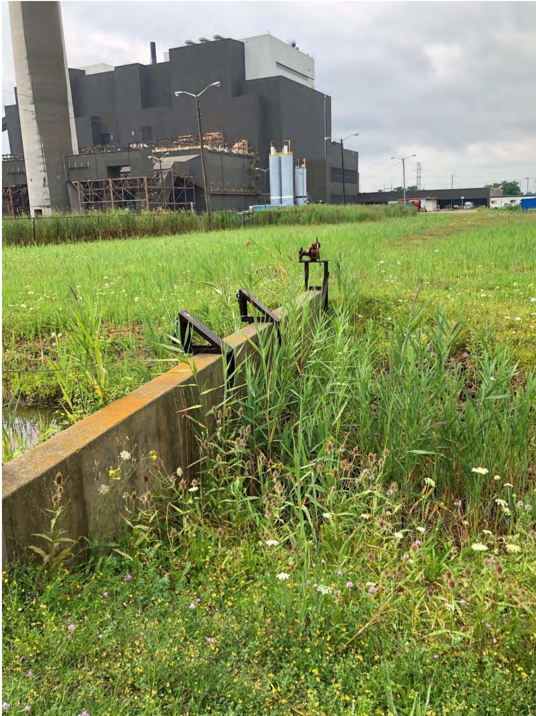
Photograph 3: Looking Approximately South from Near the Diversion Gate
