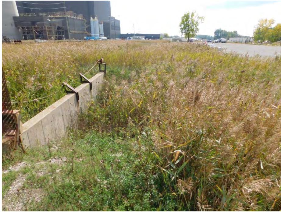
Photograph 3: Looking Approximately South from Near the Diversion Gate
