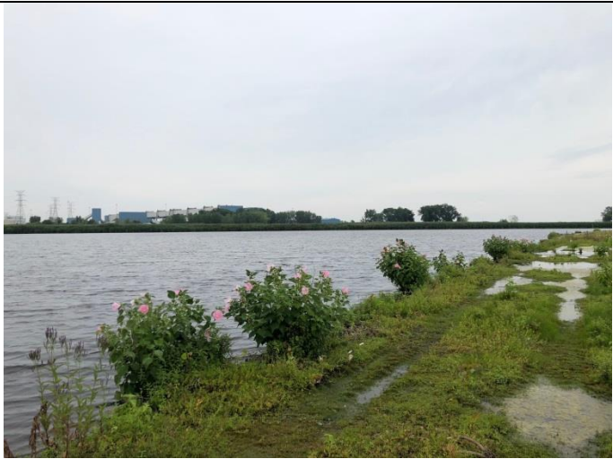
Photo 1: Looking north along east access road; note overgrown vegetation on inboard edge of berm.
