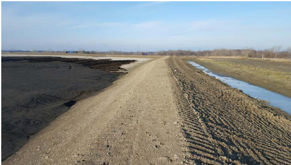
Photo 4: North Perimeter Berm near access road looking west. The perimeter swale is to the right and bottom ash is to the left in Phase 1.
