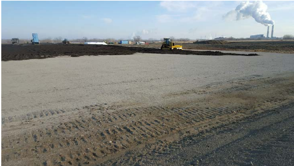
Photo 8: View of filling operations from the south berm looking northeast.
