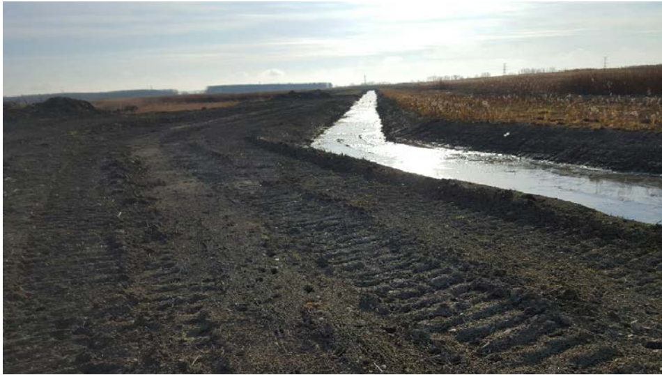
Photo 9: View of surface water drainage swale in southeast portion of the Landfill to the east of Phase 1. The Landfill construction will be to the left but has not yet reached this area.
