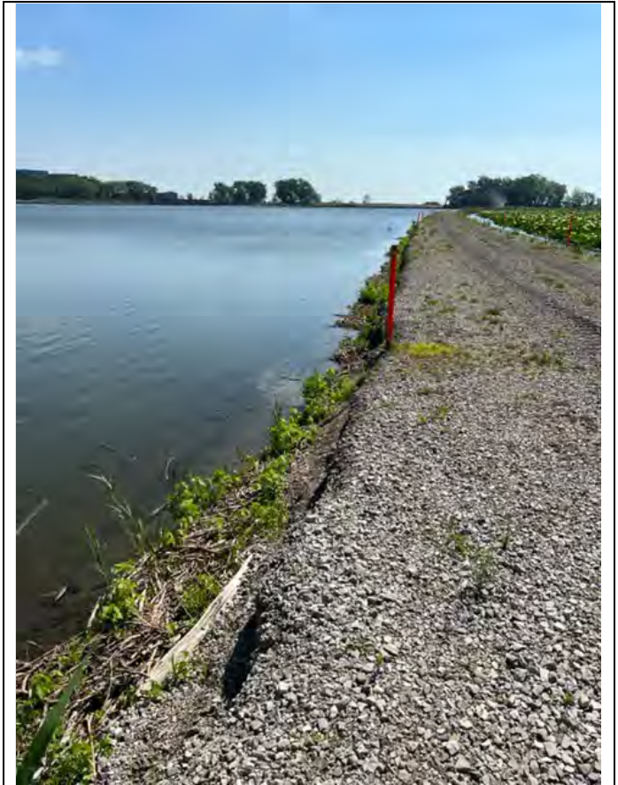
Photo 4: Another view of the southern separation berm showing the additional stone placement and sloughing along with the stable inboard slopes
