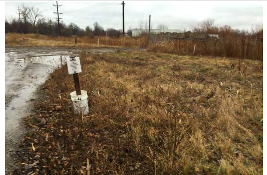
28. Gate Location Along Northeast Off-Site Groundwater Capture System. Slurry Wall Location Inside Fence at White Markers. Raining Thru-out Day.
