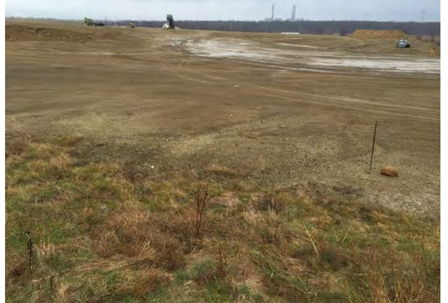
14. View of Active Portion of Phase F3 from Top of Phase F2. Ash Dry Handled Transported in Trucks Dumped and Spread.
