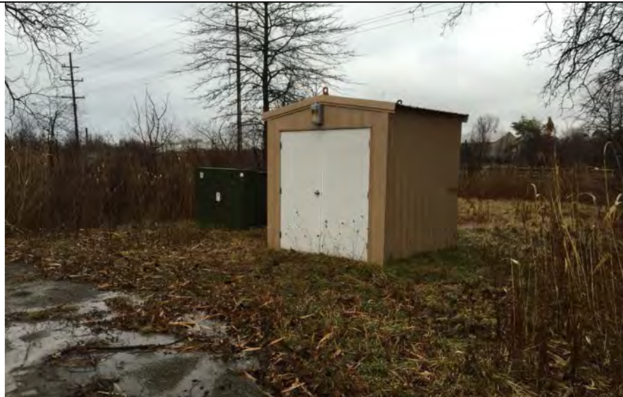
27. Northeast Off-Site Groundwater Capture System Building. Capture System Inspected Routinely and Sumps (not shown) Inspected and Cleaned 3 rd Q 2015.
