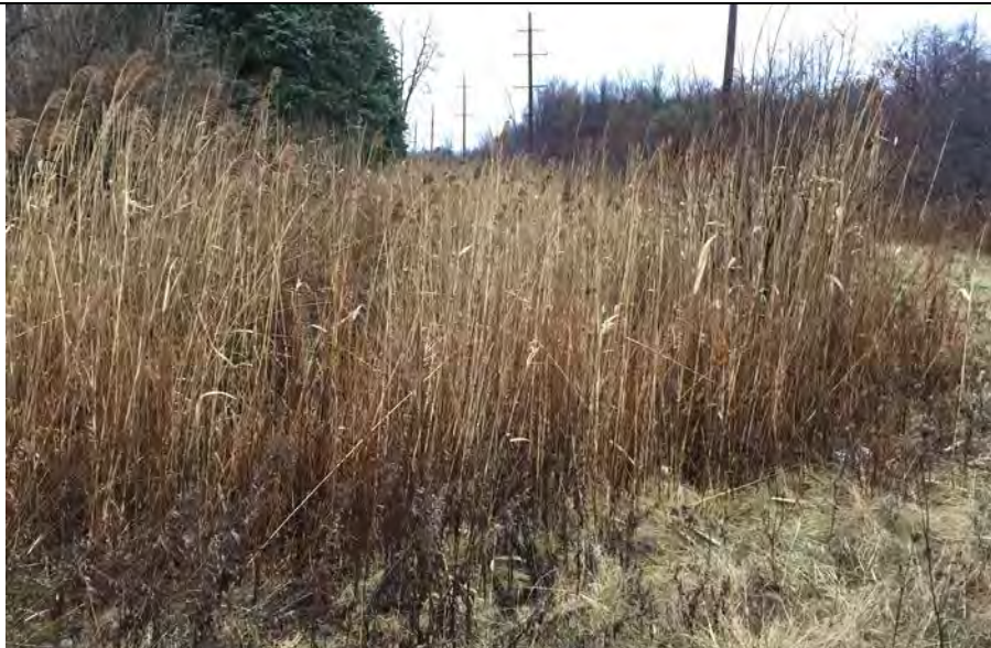
31. Perimeter Ditch Looking North from Ditch Crossing Near NE Capture System. Non-Woody Vegetation Allowed in Ditch as long as Still Flowing.
