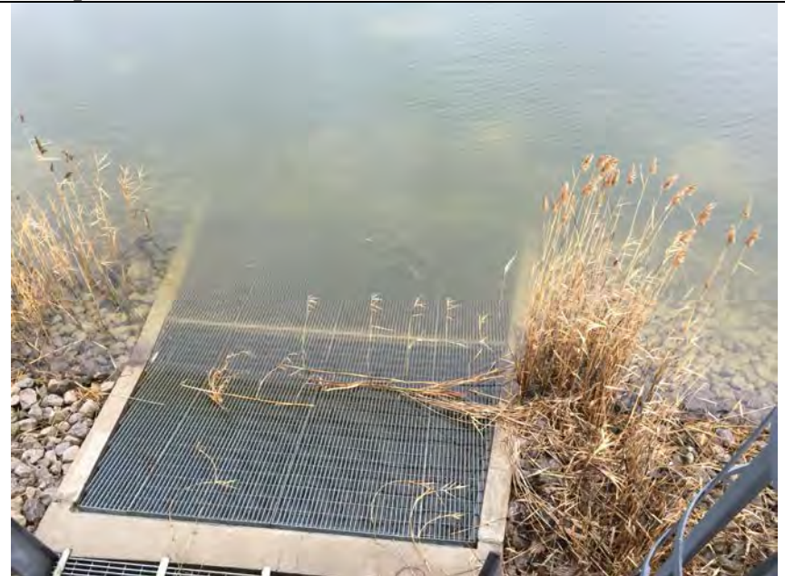
6. Basin Intake Screens. No Significant Blockage Noted.
