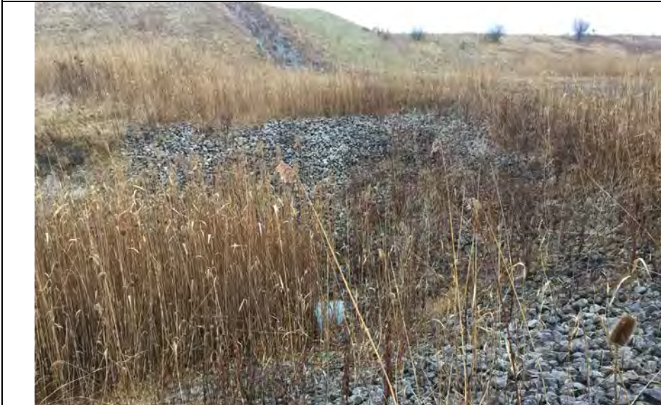
47. Construction Road Crossing of Perimeter Ditch. Culvert Shown and Stone on Slope for Surface Runoff Channel Draining to the Ditch. Runoff at Areas F1/F2 Boundary.
