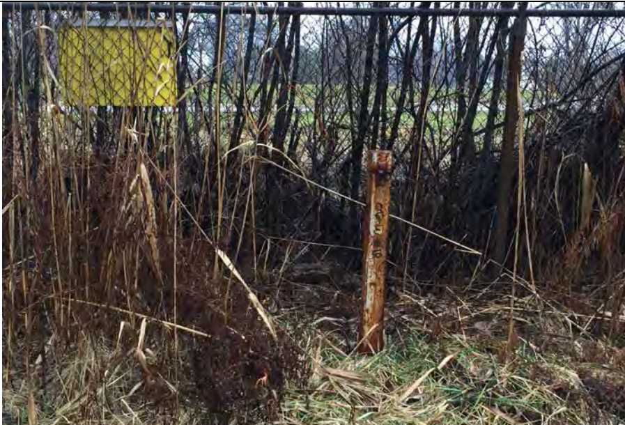
35. Observation Well or Piezometer, Believed to be OW or PZ-1R, Located Along Perimeter Property Fence Along Bree Road.
