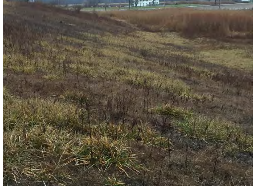
22. Close-up View of Typical Exterior Slope. Southwest Corner. Woody Vegetation on Slopes in Photos 21 - 23 and Others. Planned for Removal.
