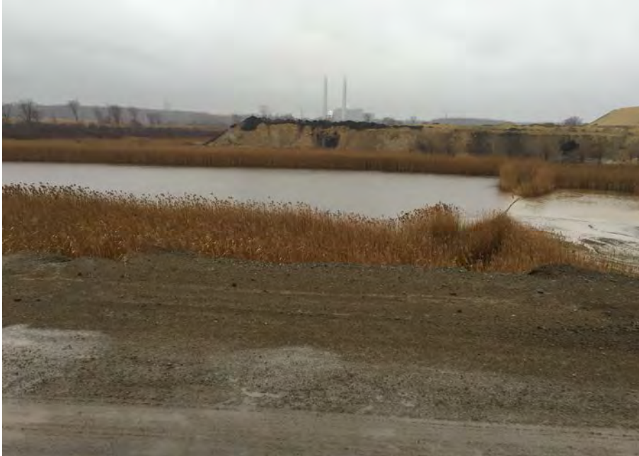
25. Runoff Collection Pond Located in Center of Landfill and Which Drains into Ditch Leading to Detention Basin.
