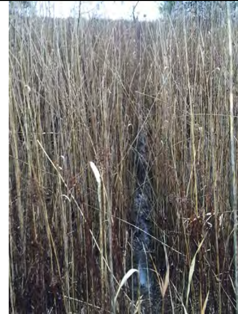
34. Perimeter Ditch Location Showing that Water is Still Flowing within Vegetation. DTE & MDEQ Allow Grassy Vegetation if Flow Maintained.
