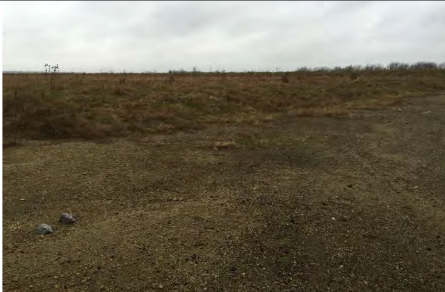
11. Top of Phase F2 Cover in Top of Photo. Phase 2 Closed in October 2012. Certification Report Viewed.
