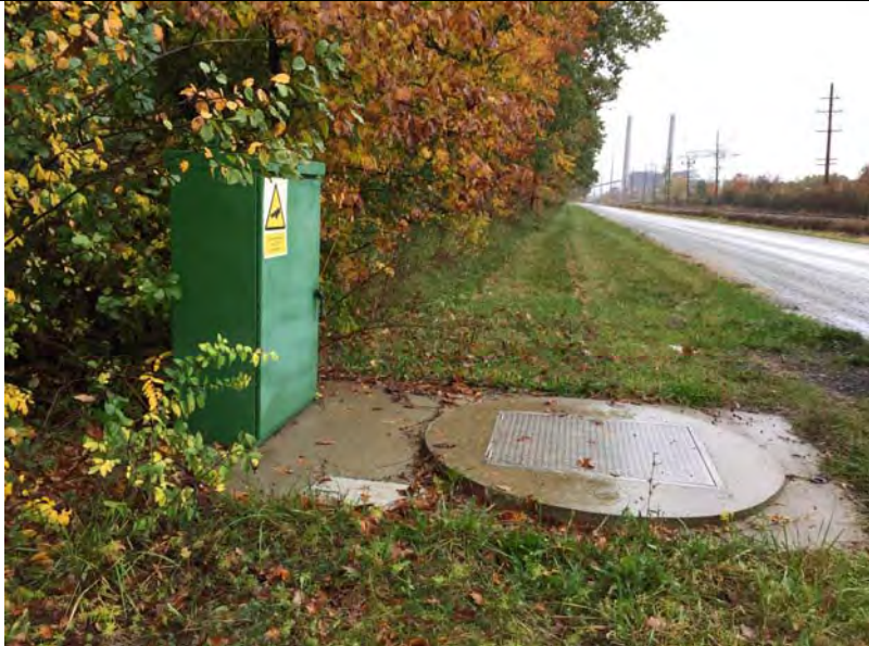
11. One of Several NE GW Capture System Sumps Located Along Range Road.
