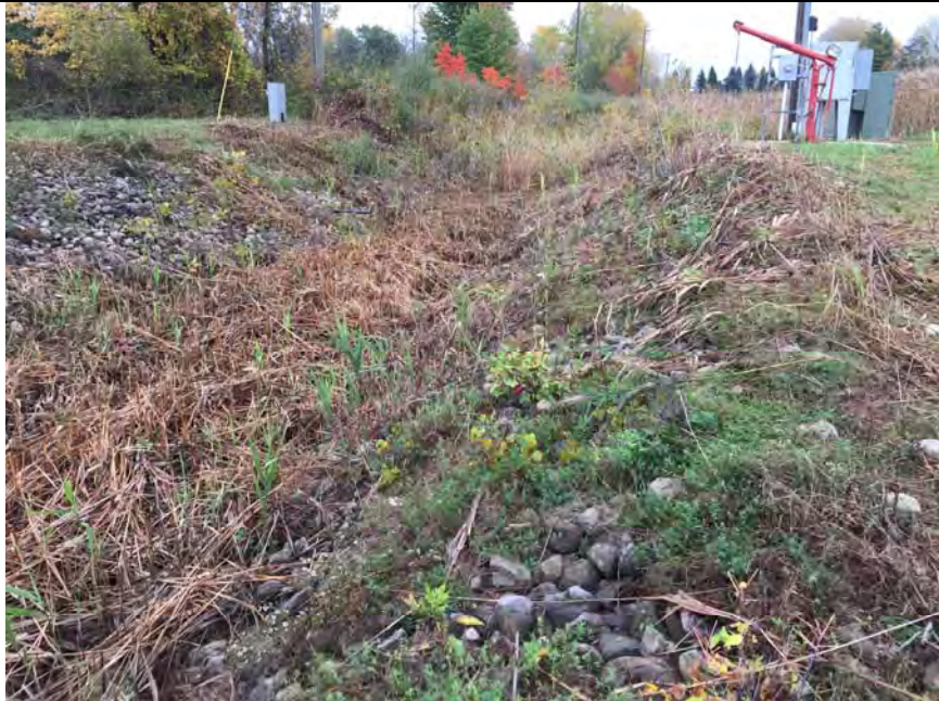
41. Perimeter Ditch Recently Cleared of Vegetation. Control Panel and Sump Location, Northwest Corner Pump Station for Offsite GW Collection System.
