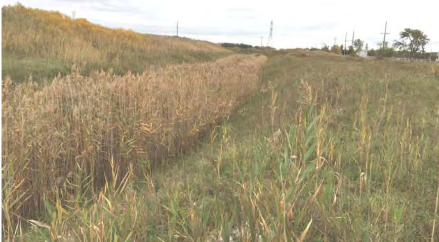
51. Looking South along SW Side at Perimeter Ditch. Vegetation has Not Blocked Ditch Flow. A 3-year Rotation Ditch Maintenance Schedule is Planned by DTE.
