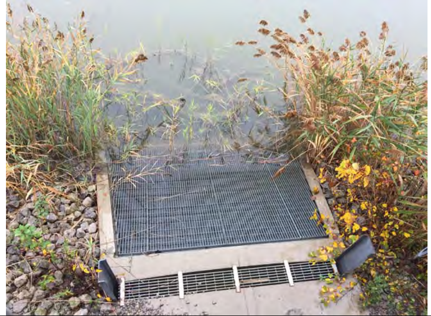
6. Basin Intake Screens. No Significant Blockage Noted.
