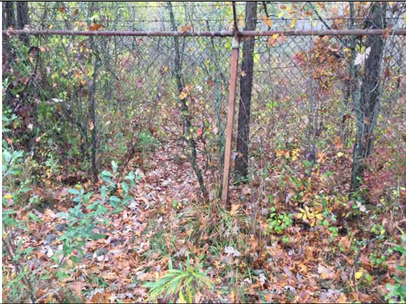
35. Small Hole in Fence At North Side Scheduled for Repair.
