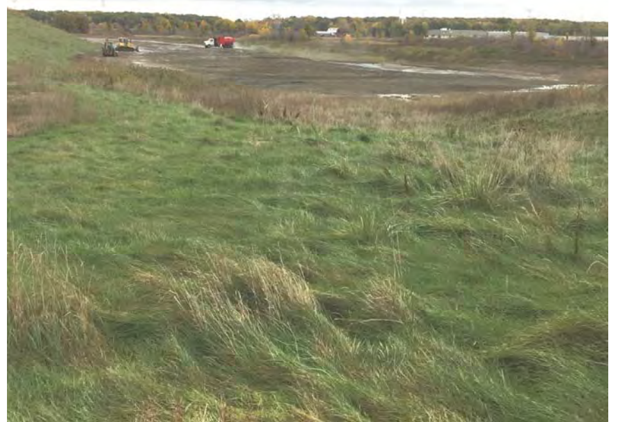
26. Looking East at the Active G2 Area Where Ash is Being Placed.
