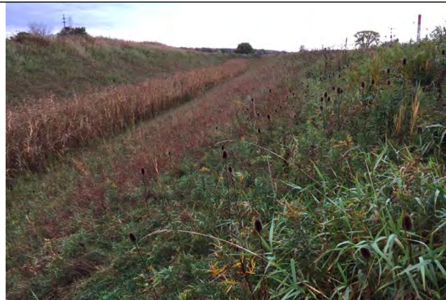
19. View of Another Portion of Reconstructed Perimeter Ditch Looking in Opposite Direction from that in Photo 18. Ditch is Open and Flowing.
