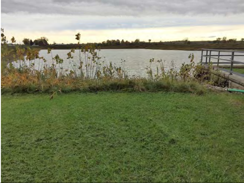
5. View of SWDB on Morning of 21 Oct. 16. Light Rain Falling.
