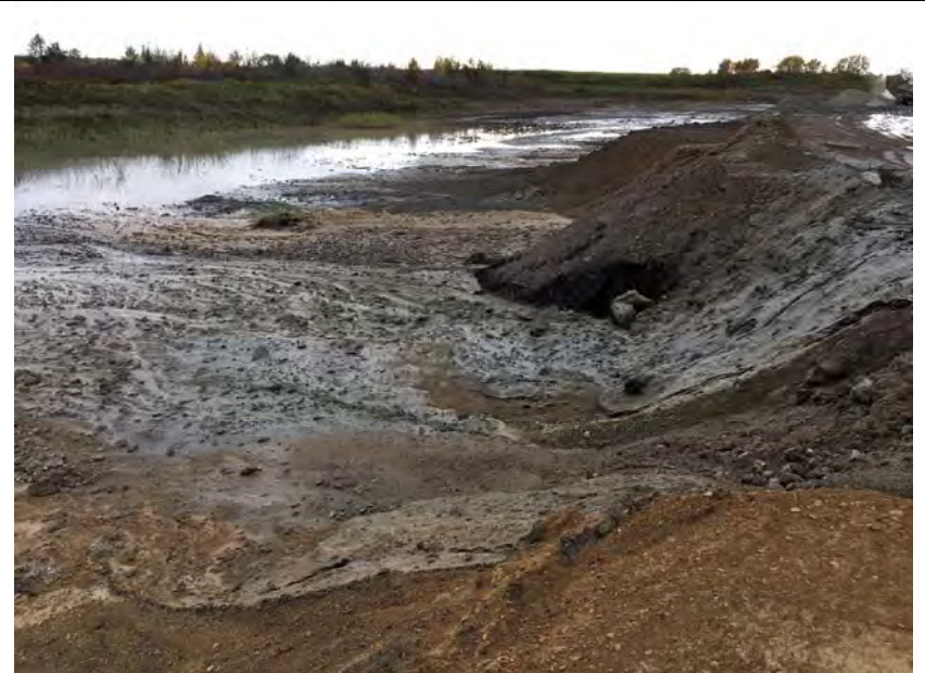
16. Water in Area G2 Drains to the Left of Photo (See Photo 15). Ash Placement In progress Far Right Corner. Heavy Rain 0.92" for 20 Oct. 16.
