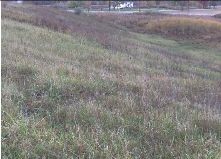
21. West Southwest d/s Side of Landfill Slope. Well Vegetated and Stable with No Significant Areas of Slope Erosion. Couple Small Woody Vegetation Noted.
