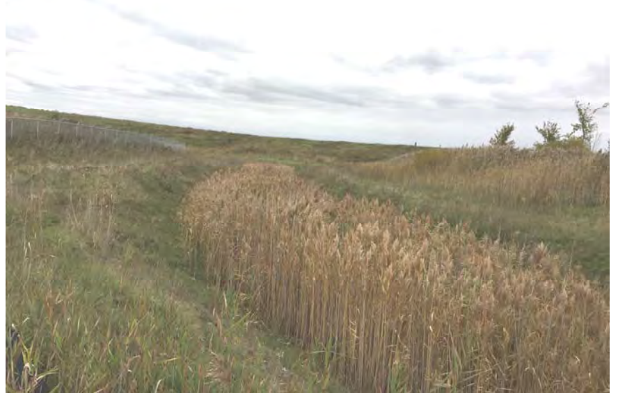
52.. Looking North at Perimeter Ditch. Ditch Slopes Appeared Stable and Well Vegetated.
