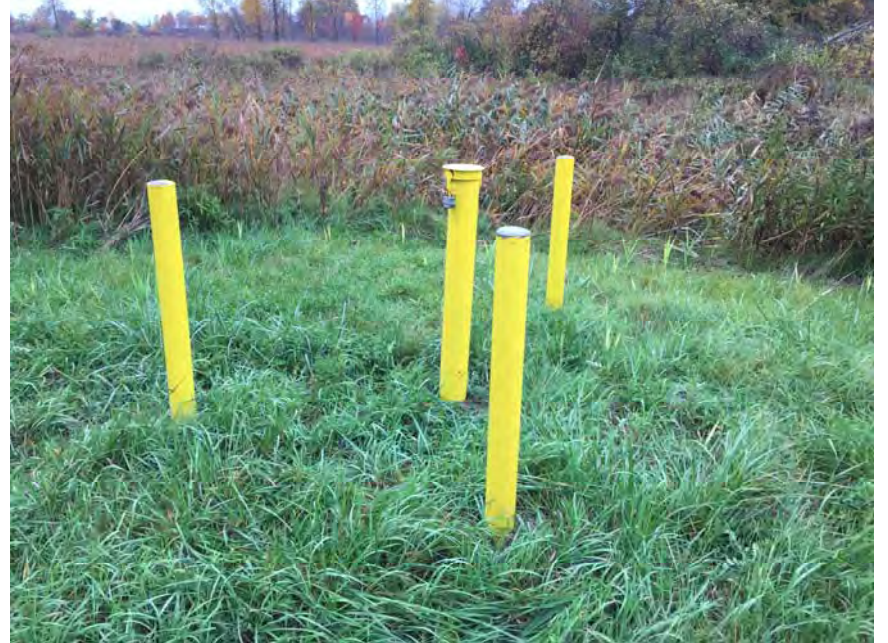
54. New CCR MW 16-02 Located East of Unconstructed Area E Near the Perimeter Ditch, but Inside of the Property Perimeter Slurry Wall.
