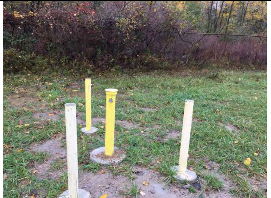
58. New CCR MW 16-06 Located Along North Side of Landfill Near Property Fence.
