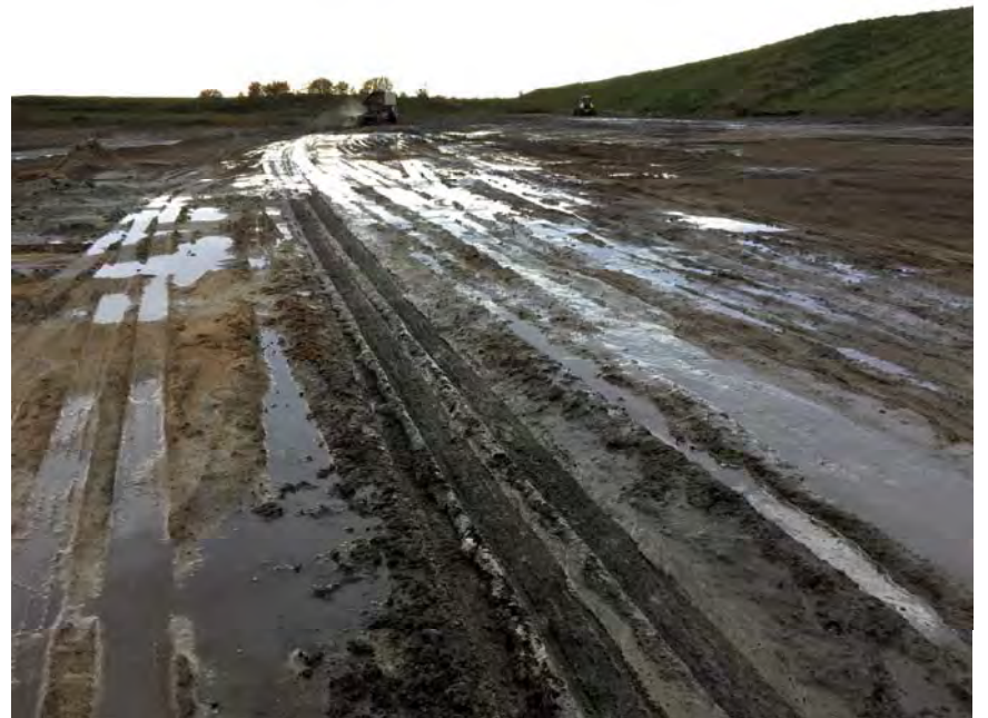
14. Active Area G2 North End. Rain Falling. Ash Being Placed at Far End Near Temporary Area F2 Slope. Little or No Tire Ruts in Ash Surface.
