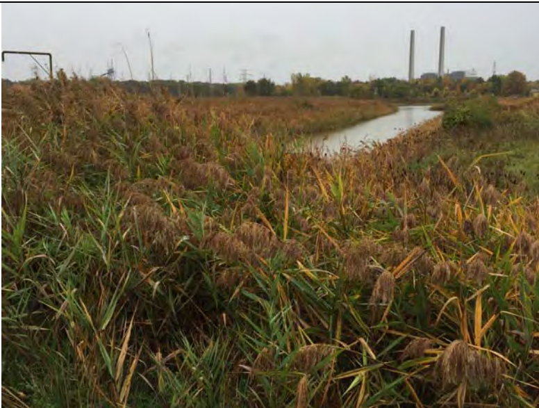
7. View of North/South Drainage Canal Leading to SWDB from Perimeter Ditch System.
