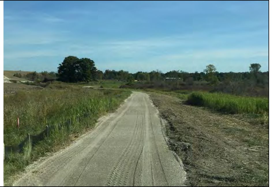
34. Reconstructed Roadway Along Perimeter Ditch on East Side.
