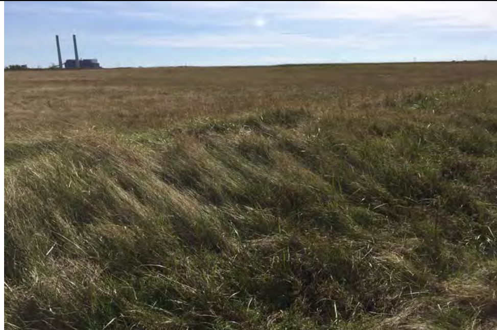
77. View of Typical Top of Closed Landfill Areas. Small Drainage Berm on Cover Shown to Contain and Direct Surface Flow.
