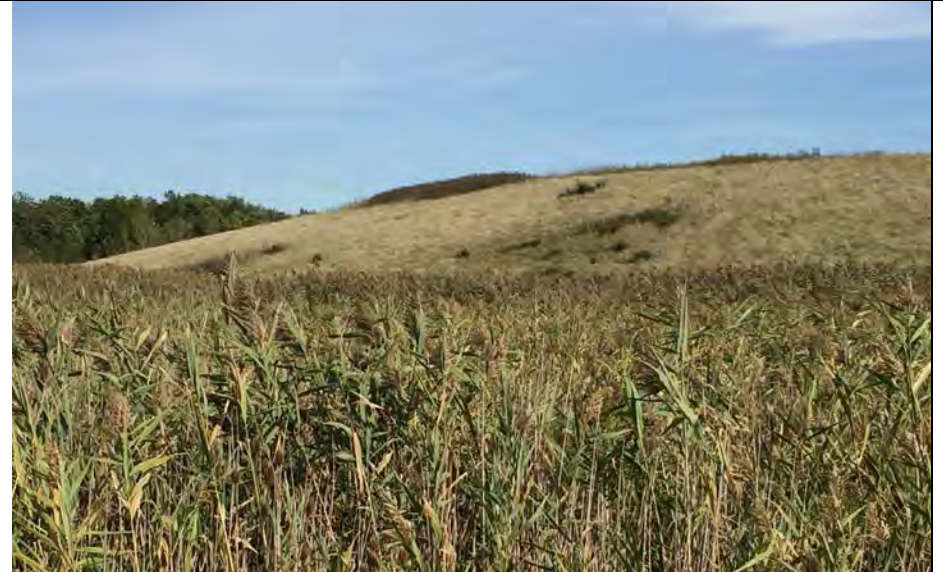
72. Looking at a Closed Area Landfill Slope.
