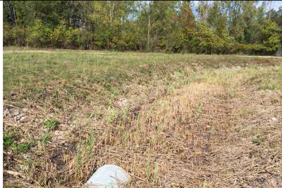
65. Area of Recent Vegetation Removal Along Perimeter East Side. Removal Equipment Observed, but Undergoing Repair or Maintenance.
