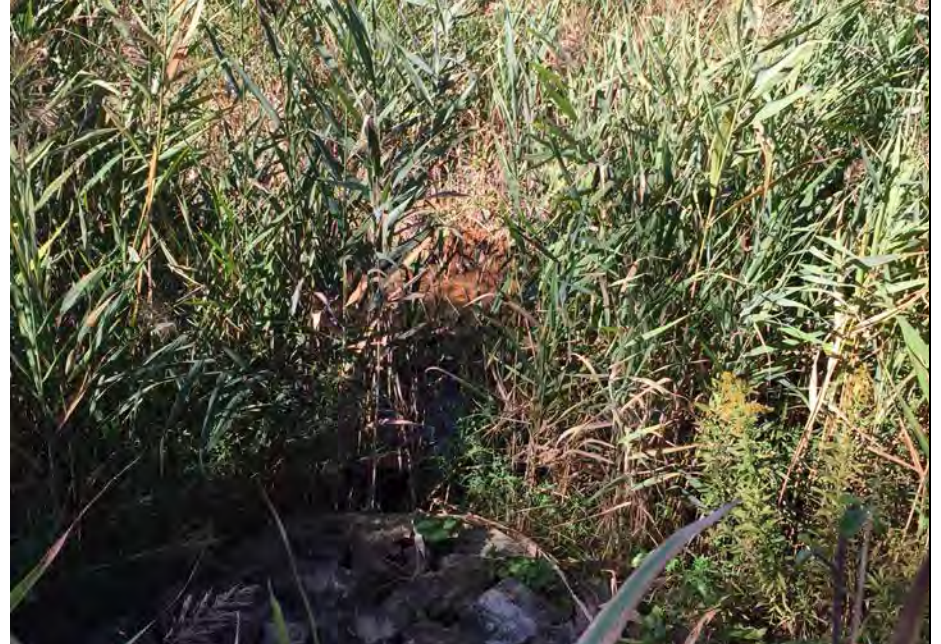
42. Discharge from Concrete Culvert into Internal Ditch. No Significant Erosion Observed.
