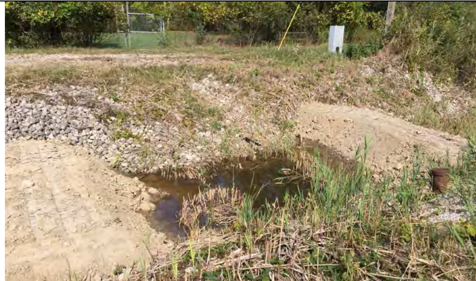
63. Collection Ditch Temporary Berms to Dam-up Water Flow.
