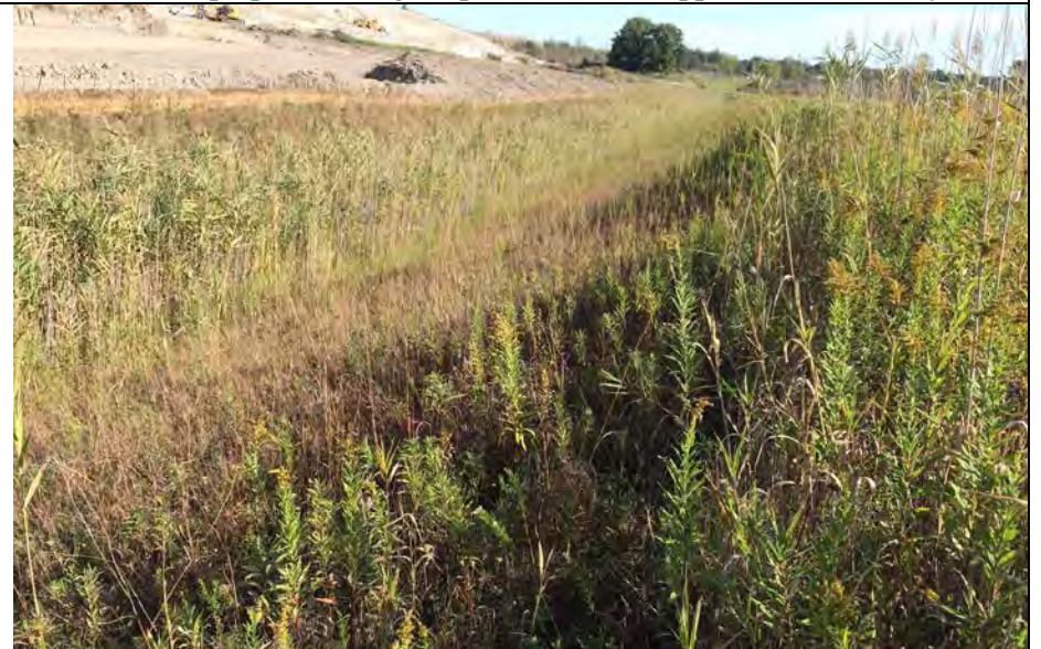
32. Internal Drainage Ditch. Vegetation Not as Heavy as Portions of the Perimeter Ditch.
