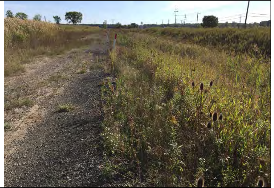
22. Looking West Along Perimeter Ditch Modified in 2010 at Right and on Alignment of Markers for Property Perimeter Installed Slurry Wall.
