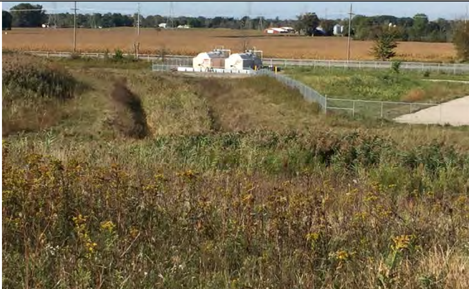
19. Looking West at Portion of Perimeter Ditch Located in the SW Quadrant of the Landfill Property. Heavy Vegetation in Bottom of Ditch.
