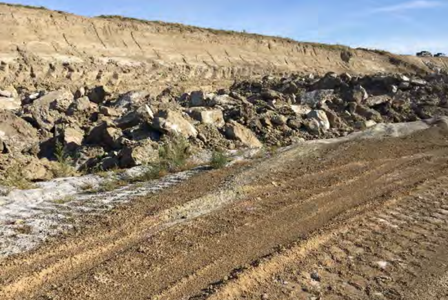
15. Looking NNE at Large Cemented Portions of Waste Removed During Removal of Interim Clay Slope on West Side of F2 Adjacent to G2 Placement.
