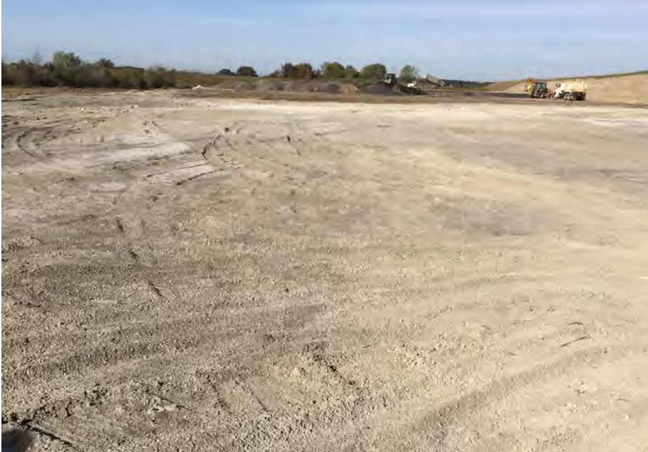
13. View Active Waste Placement Area G2 (North Side). At Top Center are Stockpiles of Dry Waste Waiting to be Spread and Compaction.
