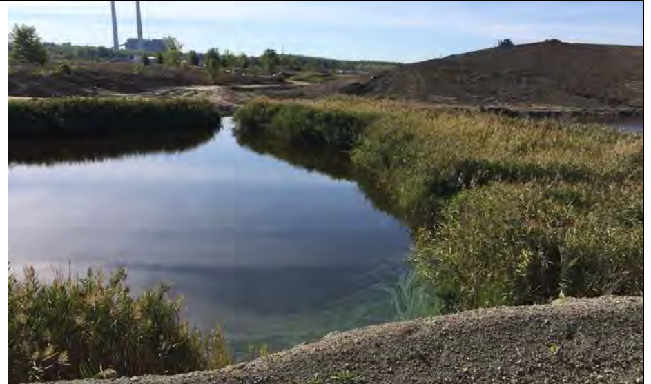
40. View of East Side of Internal Water Collection Pond.
