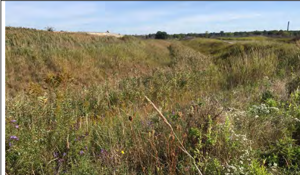
27. View of Perimeter Ditch at the SW End of Area G2. A G2 Development Survey Stake, One with Red Flags Shown, is Located at Middle of Ditch Slope.
