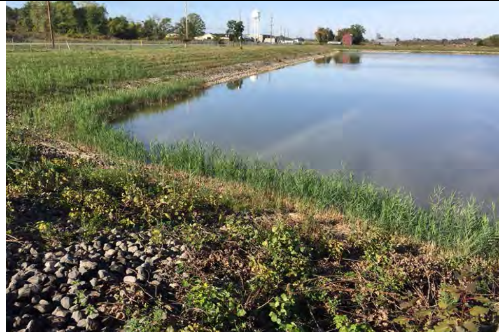
1. Storm Water Detention Basin (SWDB), South and West Sides. Slopes are Protected with Stone. No Visible Slope Erosion Vegetation Cut on Slopes.
