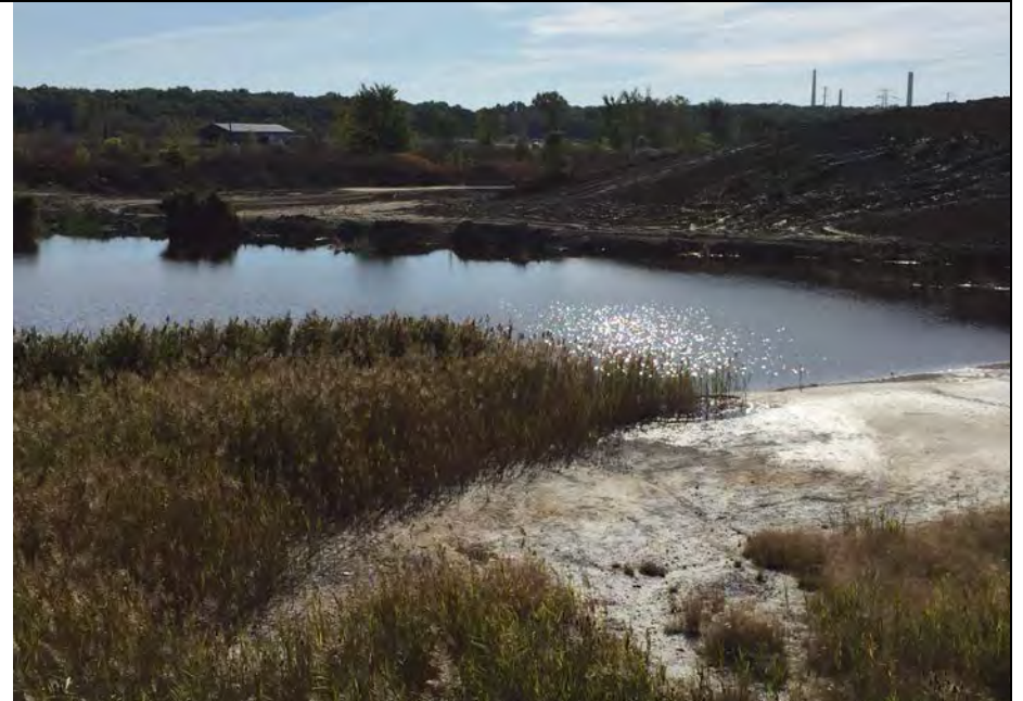
38. View of West Side of Internal Water Collection Pond Near Area F3/D3.
