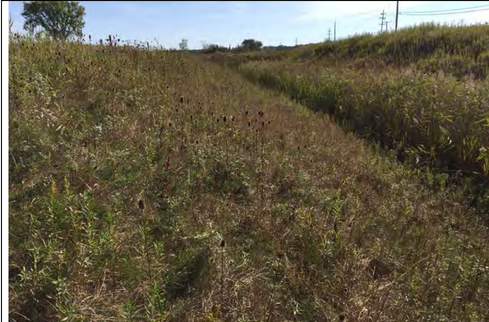
25. View of Perimeter Ditch Slopes West Side Ditch. Heavy Vegetation Bottom of Ditch. Survey Stakes Like that Shown in Photo 24 Present Middle of Slope.
