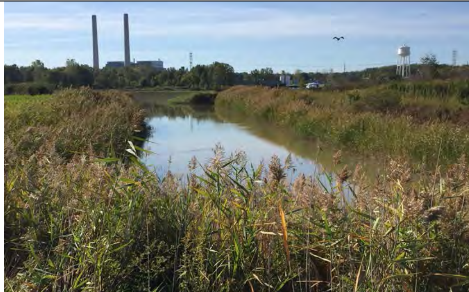
7. View of North/South Drainage Canal Leading to SWDB from Perimeter Ditch System.
