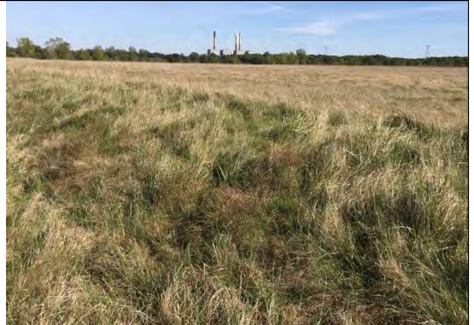
78. View of Typical Top of Closed Landfill Areas. Small Drainage Berm on Cover Shown to Contain and Direct Surface Flow.
