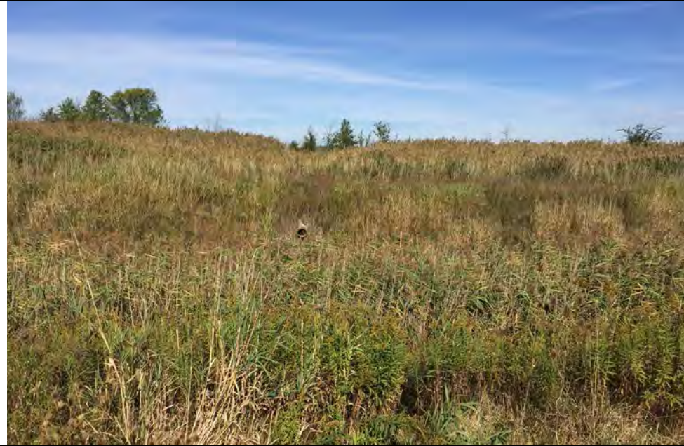
29. View of Drainage Discharge Pipe Shown in Photo 30 and Heavy Vegetation Within Perimeter Ditch.
