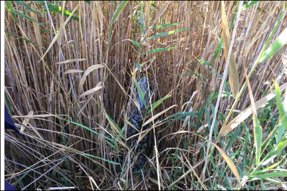
21. Perimeter Ditch View of Water Level at Bottom of Typical Heavy Vegetation Where Ditch Cleaning Has Not Occurred.
