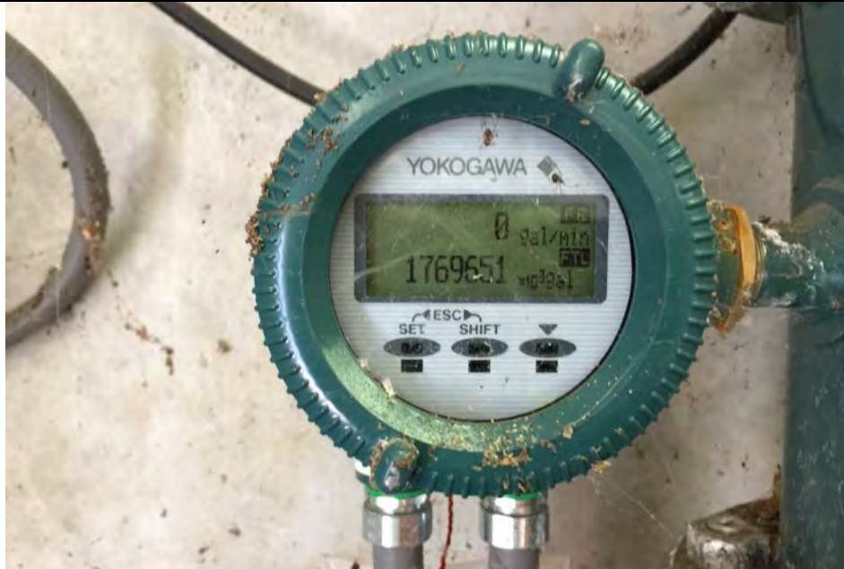
5. View of SWDB Pump Flow Meter. No Pumps On at Time of Photo, Therefore No Flow Rate Other Than "0" Shown. Total Flow Pumped is Given
