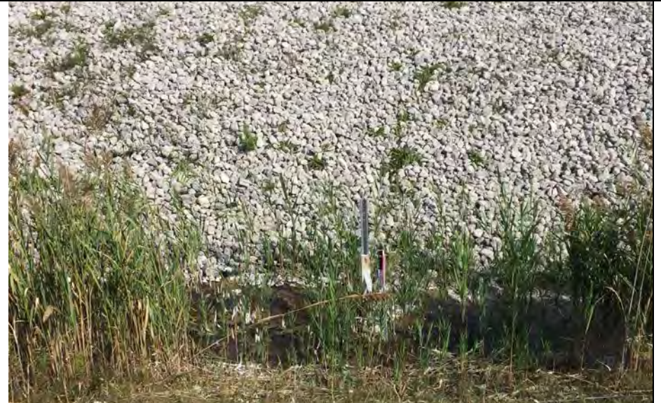
68. View of Perimeter Ditch Staff Gauge SG-09 and Stoned Slope. Gauge Not Numbered or No Longer Readable, as was Most Gauges.
