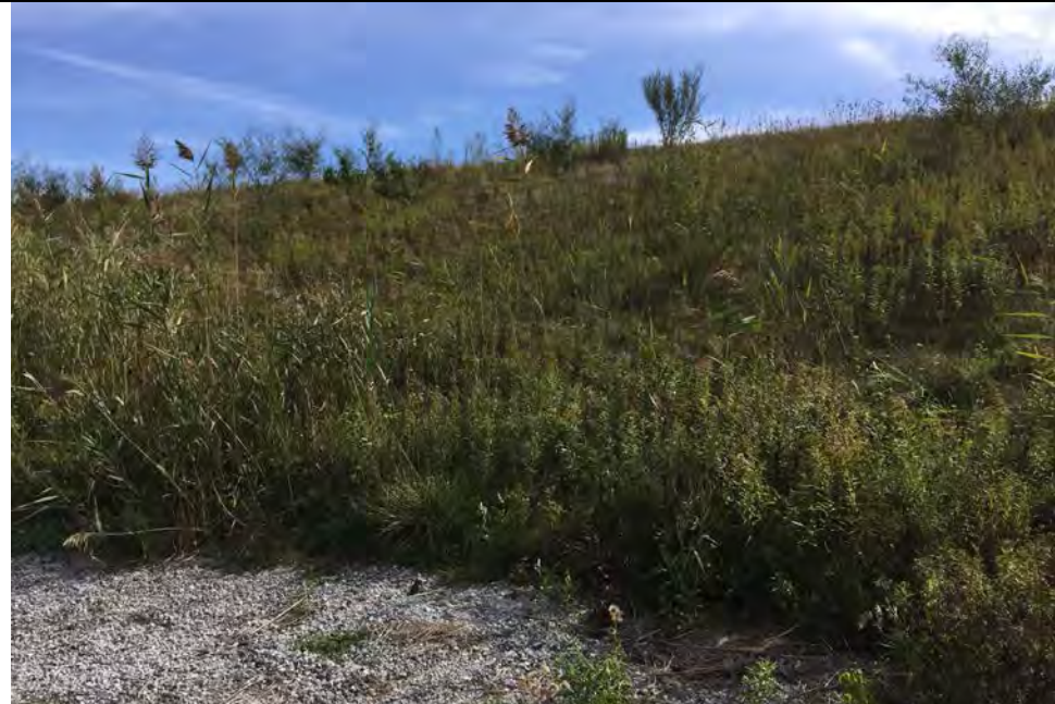
61. Brush and Small Woody Vegetation Growing on North Slope of Closed Area B of Landfill.
