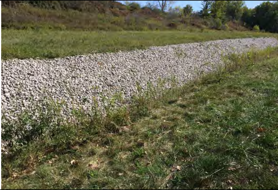
73. Looking SE at Repaired Slope of Perimeter Ditch Along West Side.
