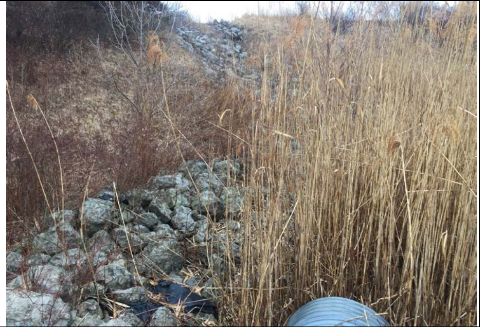
30. View of Culvert Further North at Ditch and Riprapped Downchute, both Along East Side.
