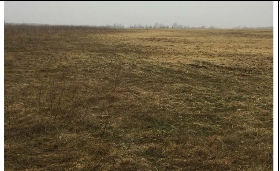
64. Another View, Left of Photo 63, of Seeded Final Cover of Area F3. No Visible Significant Surface Erosion, Although Small Tire Ruts Noted.
