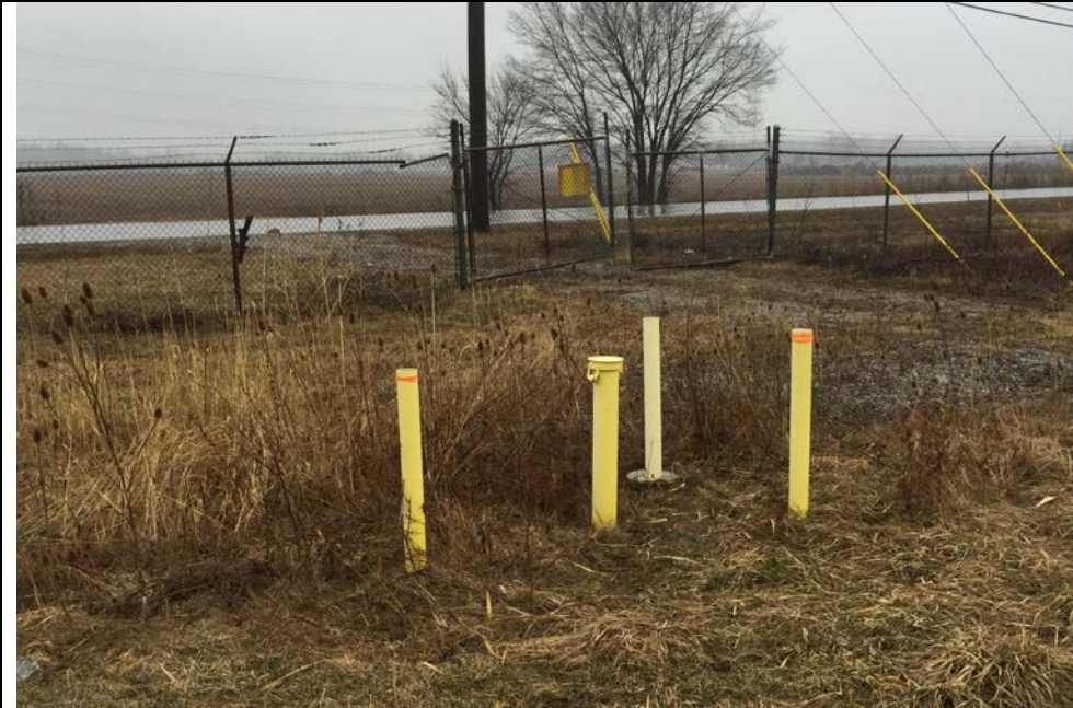
89. GW Monitoring Well 16-05 and Site Fencing and Gate Along Puttygut Road. Fence Fabric is Strung Across Chained Opening Blocking Unauthorized Entry.
