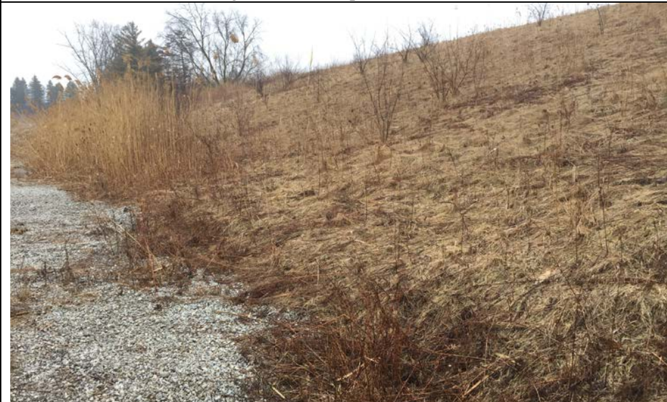
31. View of East Side Slope where Little to None Woody Tree Growth Present. Slope Uniform and Appearing Very Stable.
