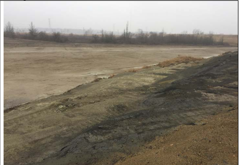
82. View of Active G2 Phase I Waste Placement Area. Bottom Area is Composed of Existing Clay Soil.
