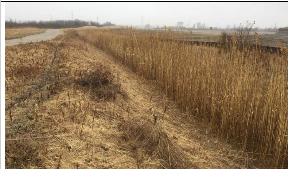
83. Landfill Perimeter Drainage Ditch at South End of Landfill. New Road Along Side of Ditch. Vegetation Cut Along Road Side. Silt Fence is Perimeter Marker of Future Area G.
