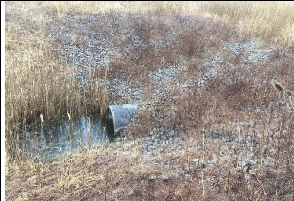
93. Upstream End of Concrete Pipe Shown in Photo 92.
