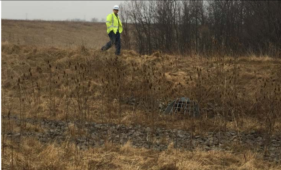
59. Landfill Surface Collection Swale Draining into Downchute Pipe. Pipe Grate Open. Bottom Slope Discharge Area of Pipe Inspected by DTE.
