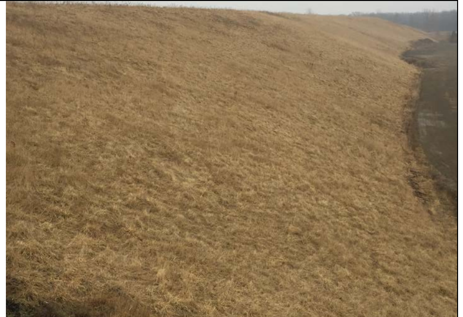
70. Another Close-up View of Slope of Closed Area D2 Shown in Photo 66. Slope Appeared Stable and Well Vegetated.
