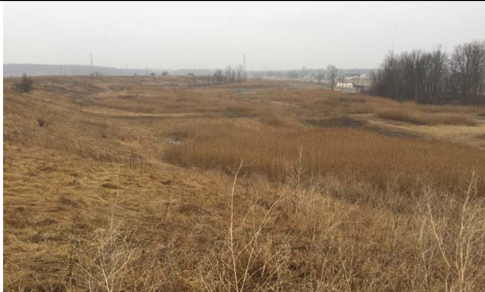
107. Looking South at West Area Outside of Landfill Storage. Landfill Lateral Drains into Perimeter Ditch Right Side of Photo. Occasional Tree Along G2 Slope to be Removed.
