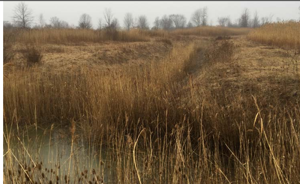
7. Looking Northeast at Drainage Ditch Draining to Canal in Photo 8. Vegetation Present, but Flow was not Blocked and Ditch Slopes Appeared Stable.
