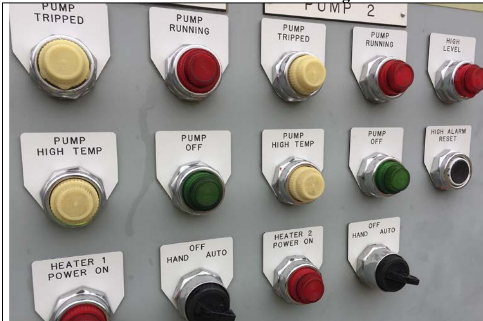
33. Control Panel at NW GW Capture System. No Pumps Currently Running, but Later Pumps were Checked for Correct Operation. Alarm Reset Cover Missing.
