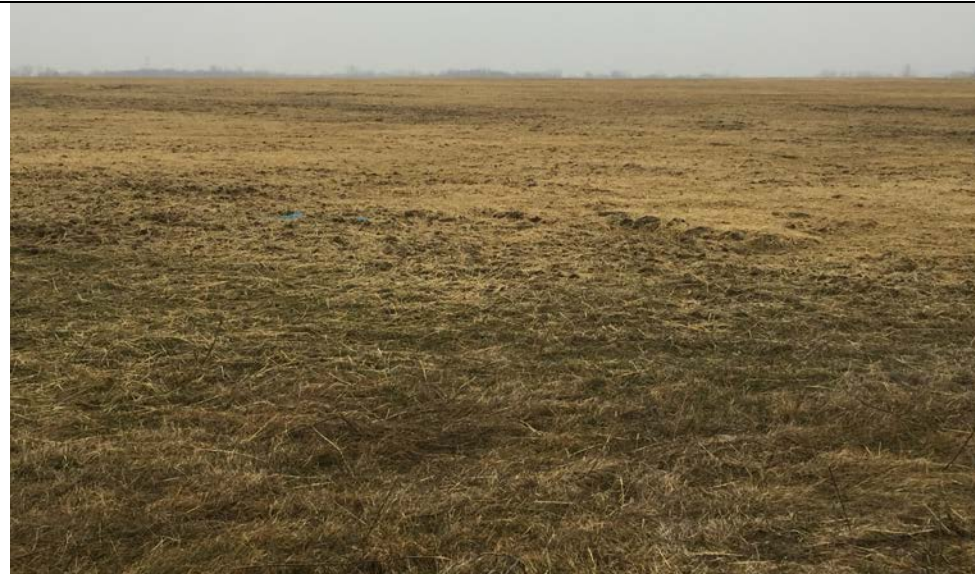
63. Another View of Seeded Final Cover of Area F3. No Visible Surface Erosion.
