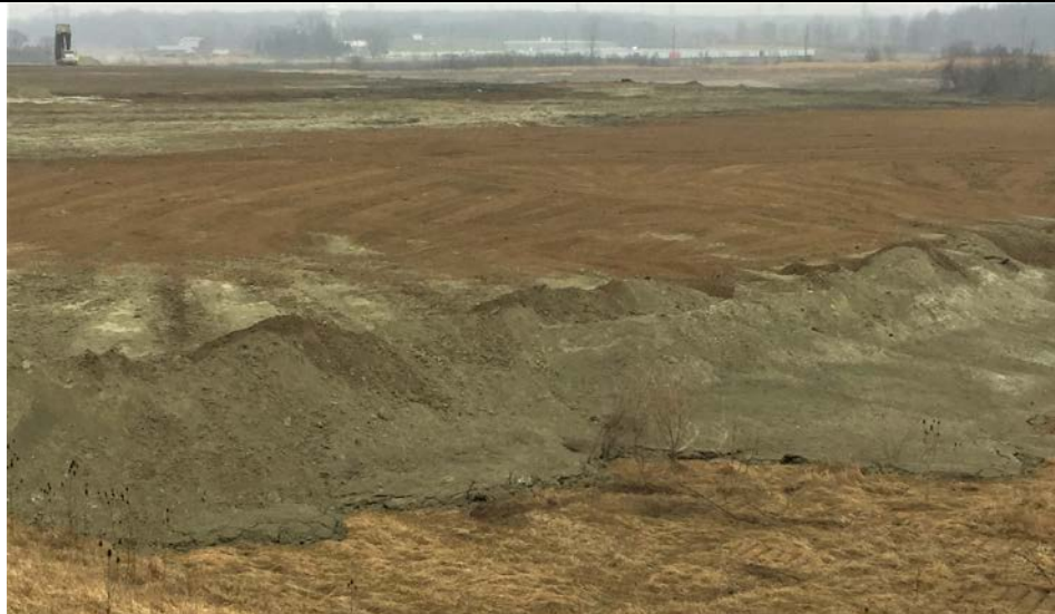
111. Waste Unloading InProgress. Piles Placed at Western Edge of Active G2 Phase 1 Area. Removal of Surface Vegetation at Western Edge Appears Not Required.
