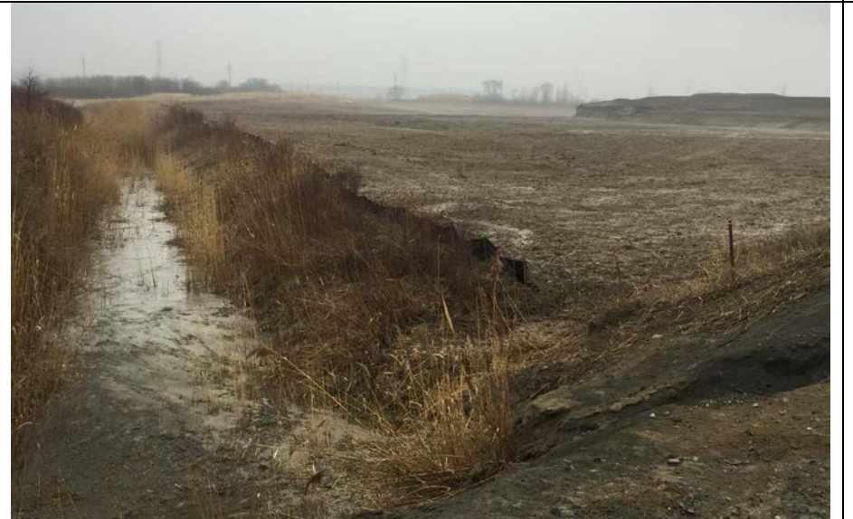
80. Old Drainage Ditch Transferring Discharge from Old Culvert.
