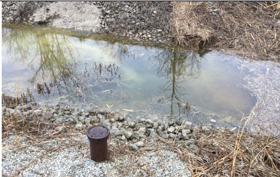
35. Collection Ditch and Intake to Sump at NW Groundwater Capture System. Vegetation Debris was Removed at Intake to Increase Flow to Sump.
