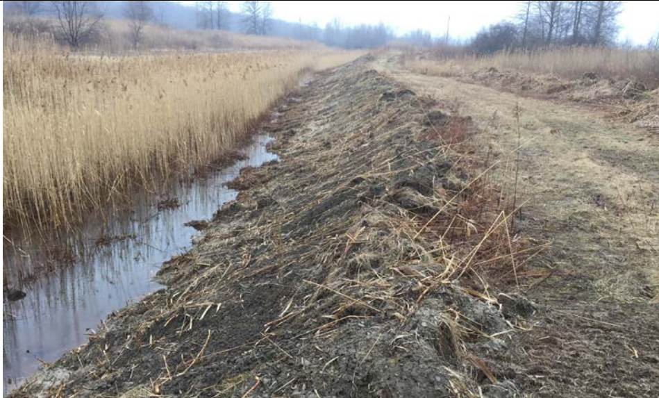
75. Ditch Maintenance Clearing Vegetation and Flow Grades.
