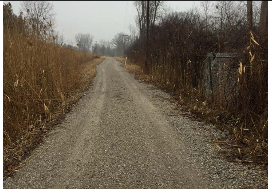
26. View of Perimeter Road Left Side Ditch. Road was Up-graded Making Maintenance/Monitoring More Accessible. Slurry Wall Marker Shown.
