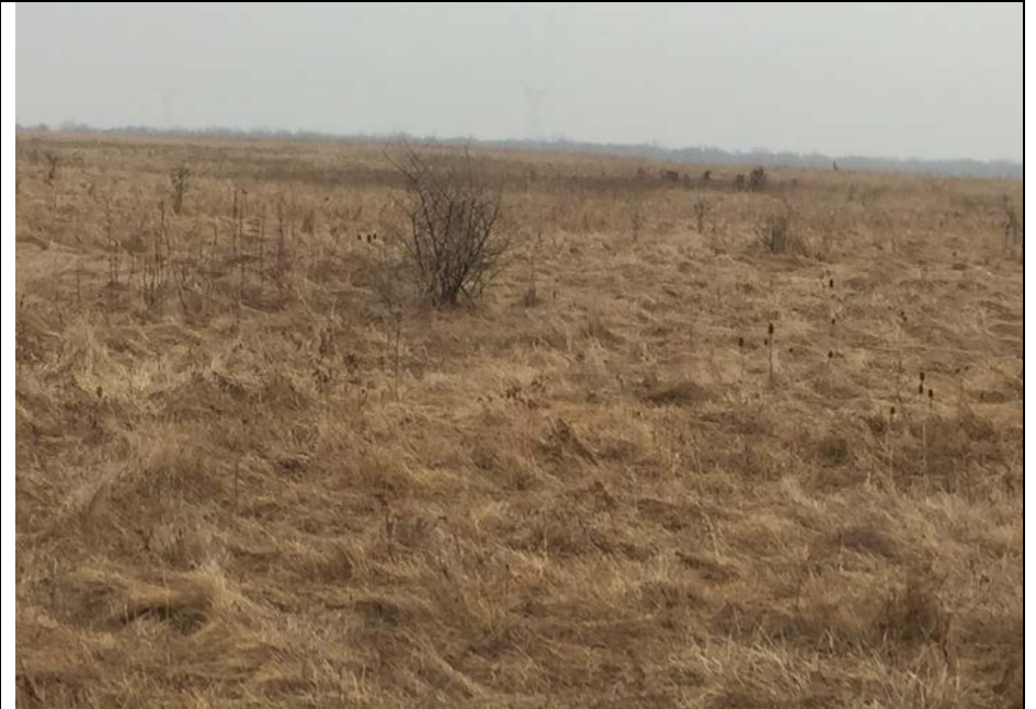
58. View of Top of a Closed Landfill Area Containing Some Minor Small Woody Vegetation. Top Well Vegetated and Free of Erosion.
