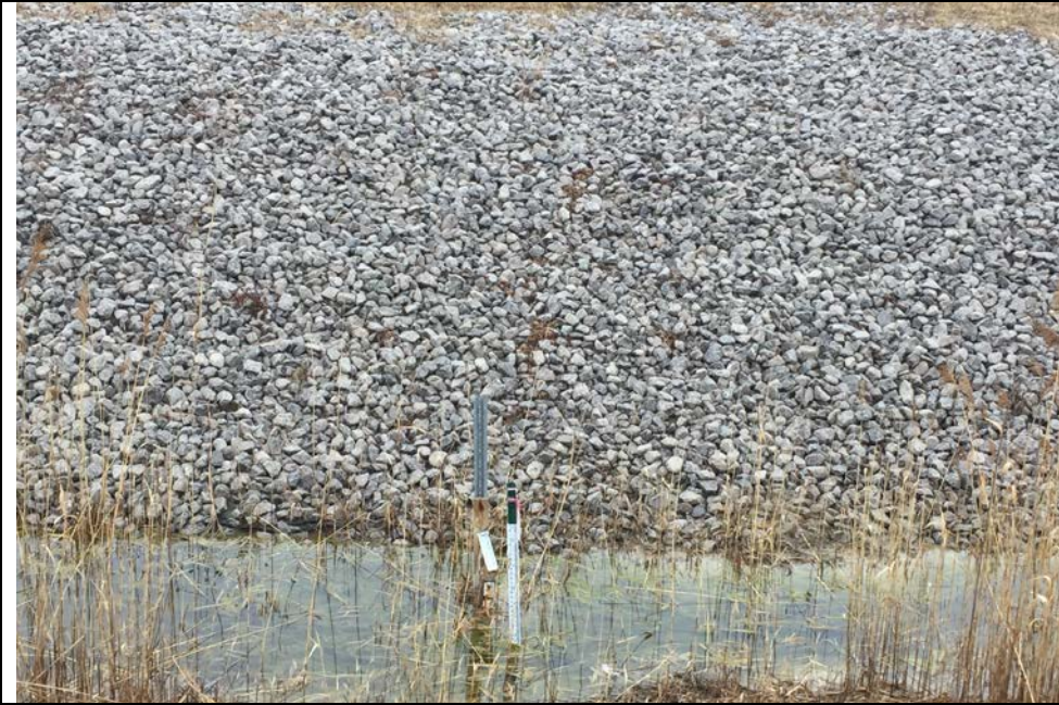
45. View of Stoned Slope and Staff Gauge SG-09 Located West Side of Closed Area F1.
