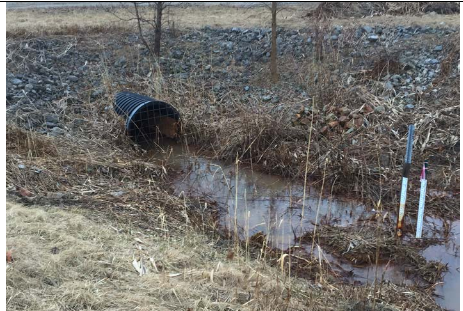
16. Closeup View of Culvert at Crossing and Staff Gauge SG-5.
