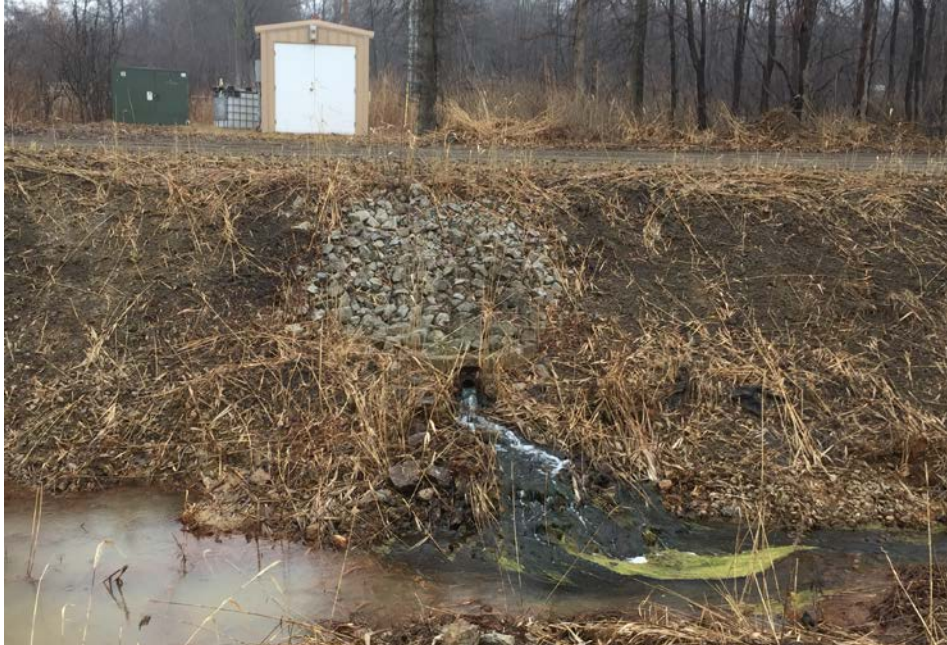
13. View of Discharge Flow into Perimeter Ditch from NE Off-Site GW Capture System at 11:47AM. Also Ditch Slope Vegetation Cleared Late Last Year
