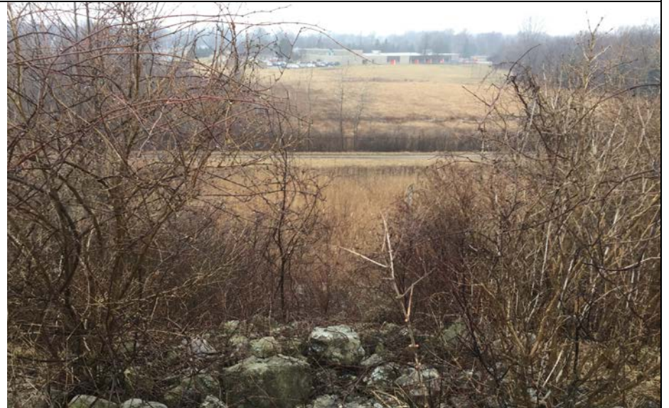
56. Looking Downslope at Downchute of North Slope of Closed Area B.
