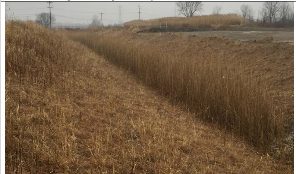
87. Looking Southwest at Perimeter Ditch at West Side of Area G2. Ditch Slopes Appeared Stable and Well Vegetated. Slope Vegetation Cut Late 2017 or Early 2018.
