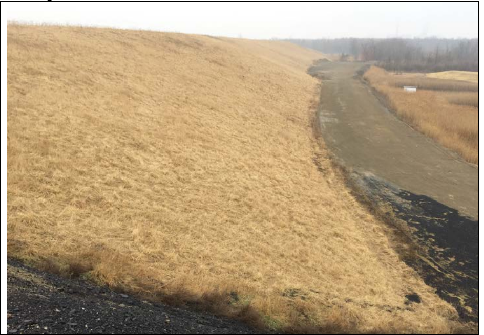
66. Looking North at Slope of Closed Area D2. Slope Appears Stable and Well Vegetated.
