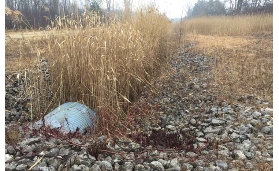
28. View of Culvert and Perimeter Ditch with Heavy Bottom Ditch Vegetation.
