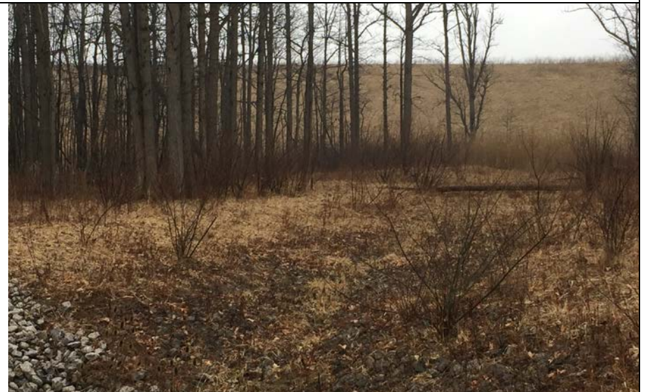
44. Vegetated Landfill Slope West Side of Area B. Lateral Ditch Draining Downstream Area. No Visible Slope Stability Problems.
