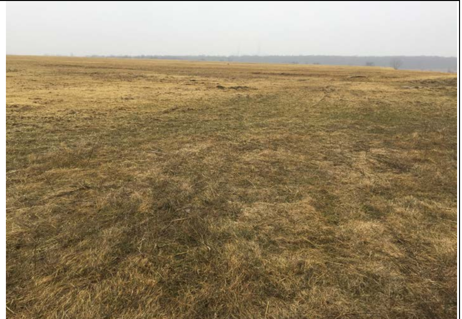
62. Looking NE from Closed Area F2 at Southeast Side of Seeded Final Cover of Area F3. Seeding Completed Late in 2017,
