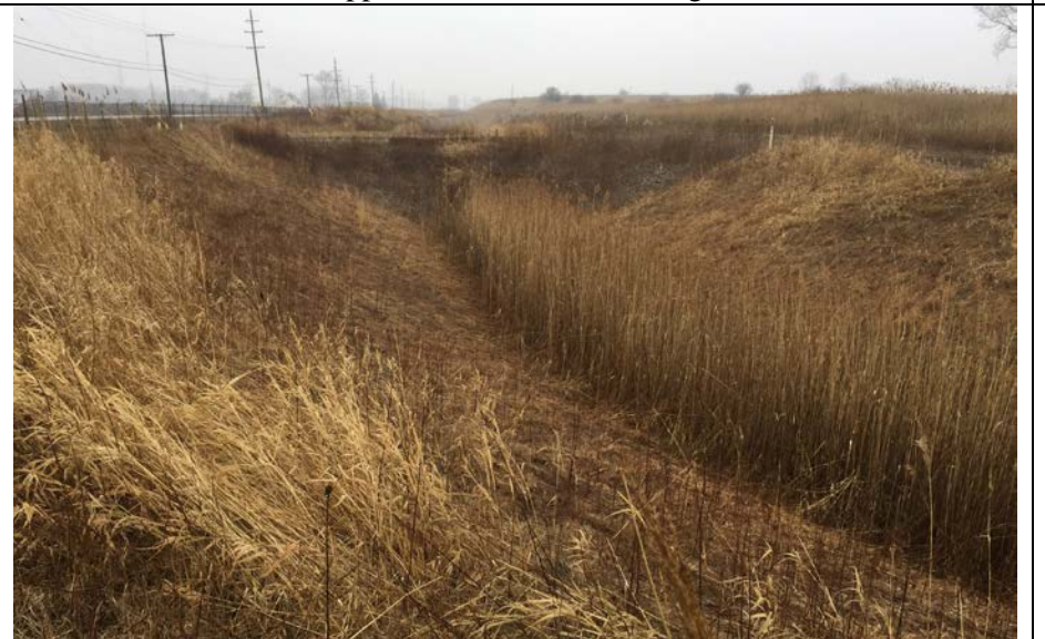
88. Looking West at Perimeter Ditch. Slope Vegetation Has been Cut and Slopes Appear Stable and Well Vegetated. Site Road Crosses Ditch at Top.
