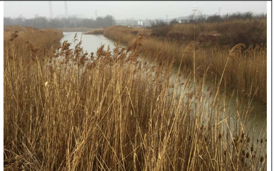
8. View of North/South Drainage Canal Leading to SWDB from Perimeter Ditch System.
