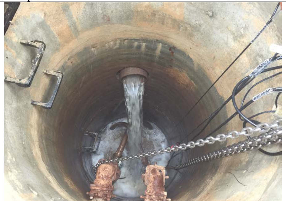
34. Sump Showing Increased Flow from Collection Ditch (See Photo 35) after Blocking Vegetation Removed by DTE During Inspection.
