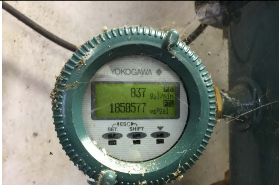
5. View of SWDB Pump Flow Meter. One Pump On at Time of Photo, Therefore Flow Rate Shown at 837 gal/min. Total Flow Pumped is Given.
