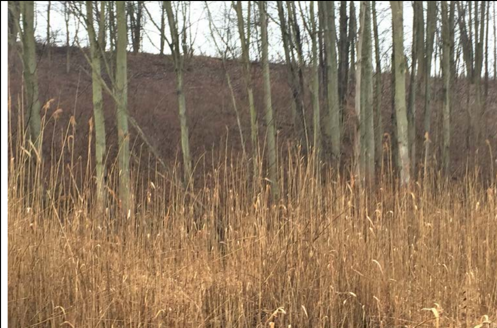
41. Tree Growth Heavy Along Closed Landfill Toe, Less on Slope. No Stability or Erosion Problems Noted on Slope. Top of Slope Inspected Later in Day.
