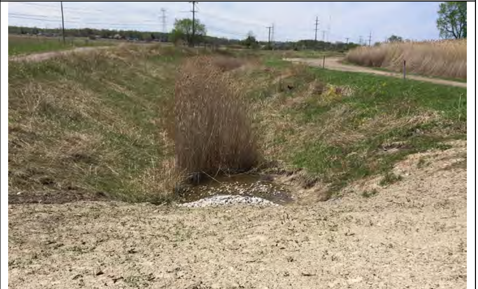
44. Perimeter Ditch South Side. Some Bottom Vegetation but No Flow Blockage.
