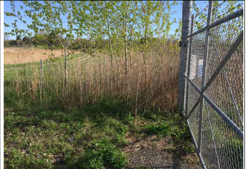
10. Side View of Locked Gate with Signage and at Far-Left Typical Slurry Wall Location Marker. All Gates had Signage.
