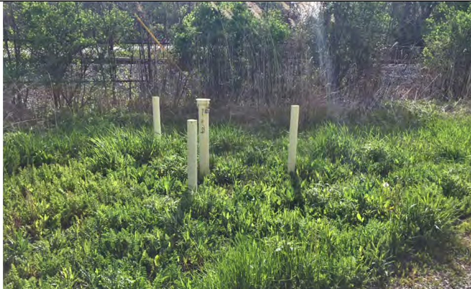
7. Monitoring Well 16-04. Well Protected and Cap Locked. Well Protection and Capping Typical of Inspected Above Ground Monitoring Wells.
