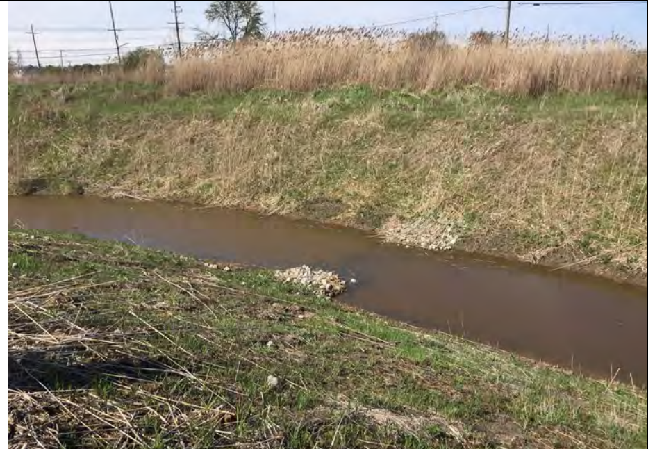
26. Perimeter Ditch Southwest Side. Check Dam Shown. No Ditch Blockage.
