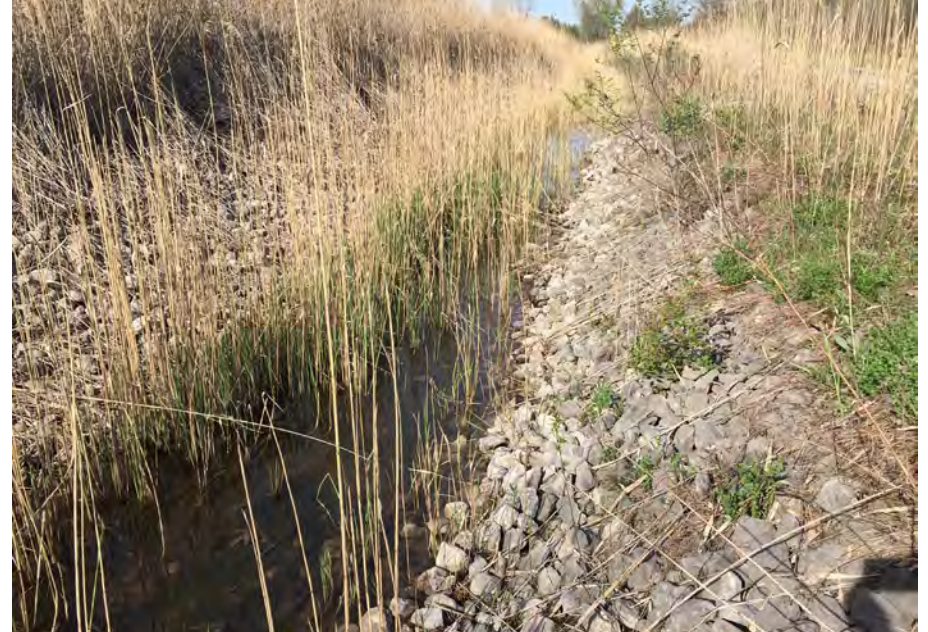
18. Looking at Portion of Perimeter Ditch Alignment Cleared of Vegetation Last March. Little Flow Noted.
