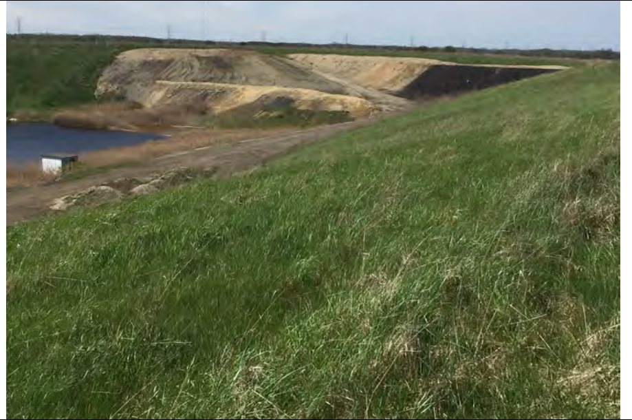
36. Right side of runoff collection pond within landfill limits. Area F3D3 in corner where road ramps shown to top of landfill.
