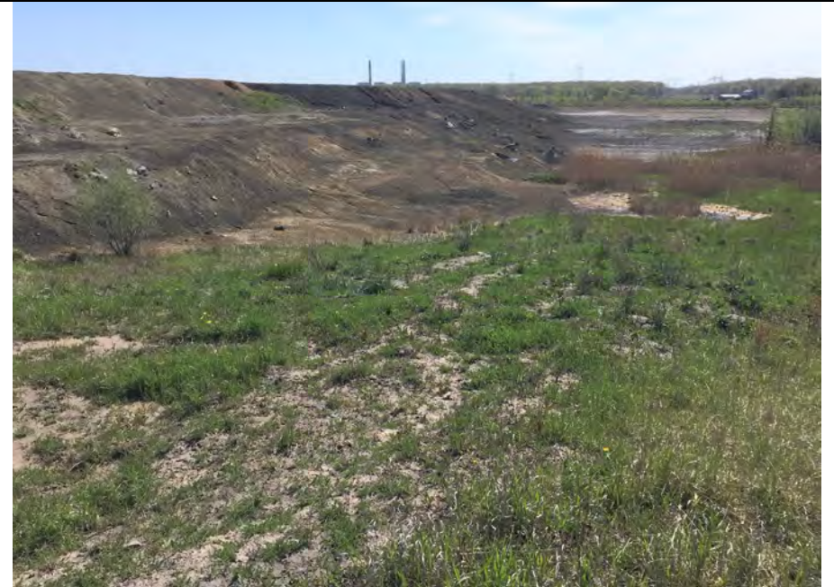
30. Continuation of Photo 29 as Top of Area F2 Slope Meets Portion of Area G2 Approved for CCR Disposal.
