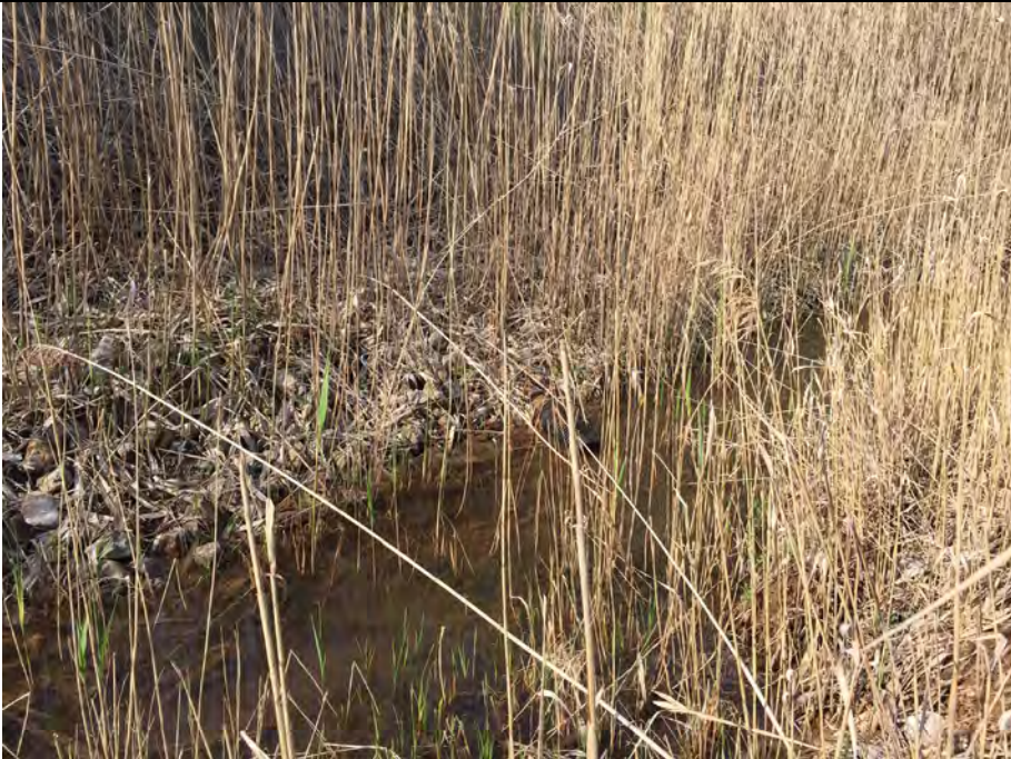
21. Looking at Perimeter Ditch North Side of Landfill. At Photo Center is Black Corrugated Pipe Likely Collecting Slope or Gully Drainage. About 6 Noted.
