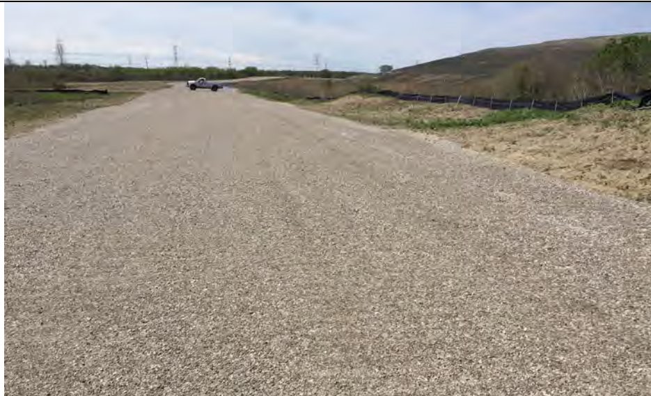
43. Newly Constructed Interior Landfill Haul Road.
