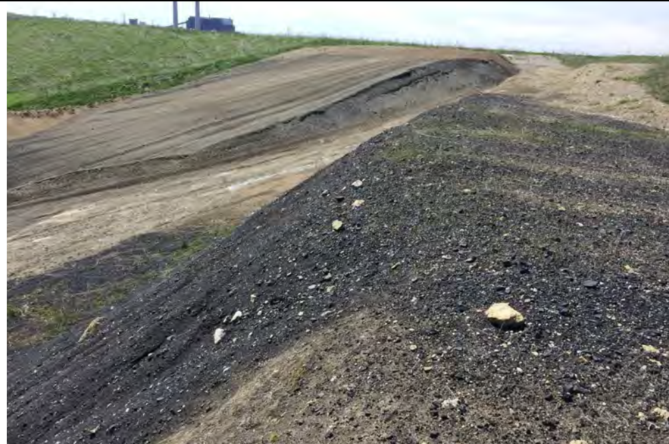
37. Interior Haul Road Leading Down into Active Waste Placement Areas. Compacted Waste Supporting Haul Trucks Without Rutting.
