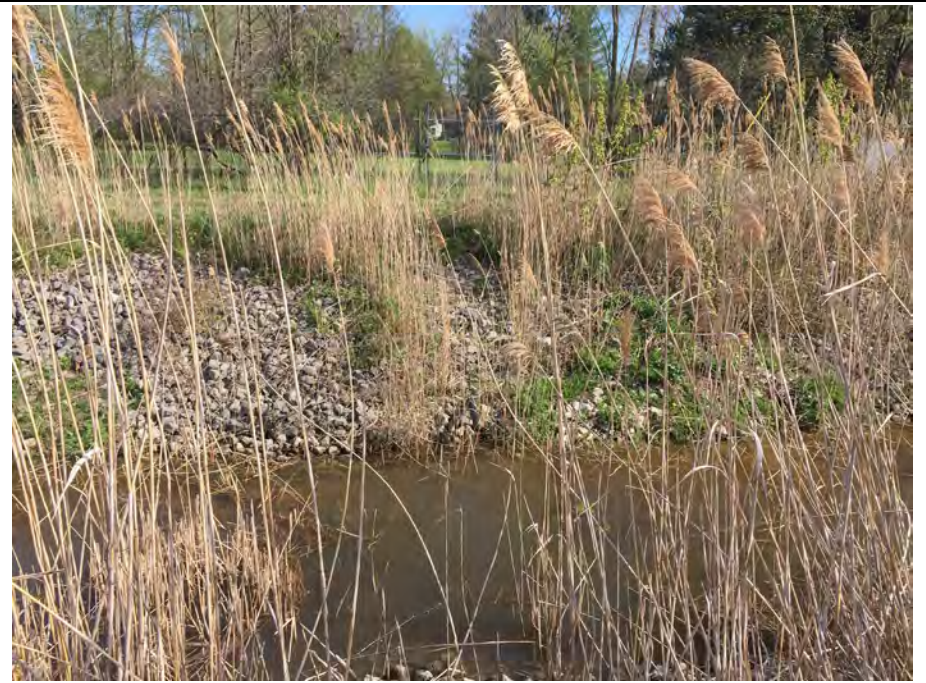
22. Location of Discharge Pipe from Offsite GW Capture Area. Locked Gate in Background Easily Noticed in Photo when Zoomed in.
