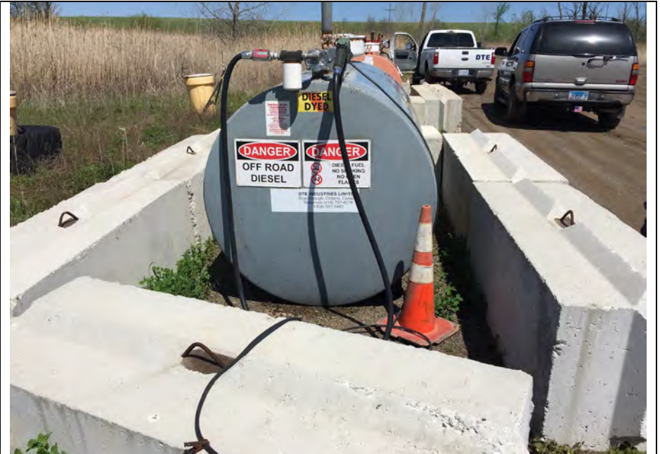
42. Looking at First Fuel Tank and Protection Containment and Signage.
