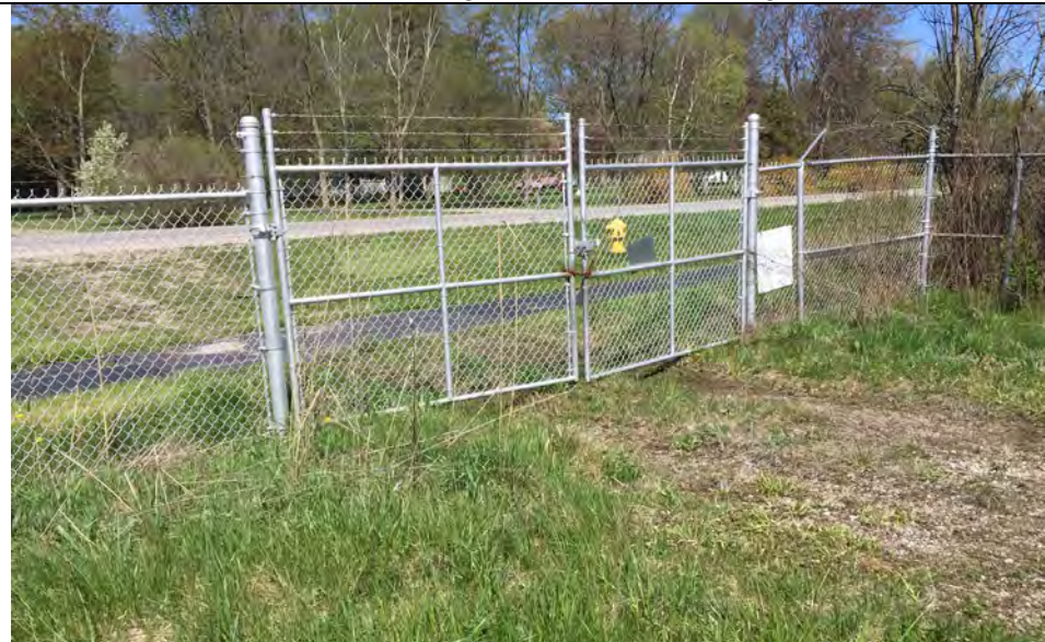
31. Northwest Corner Fence and Locked Gate, Signs Posted.
