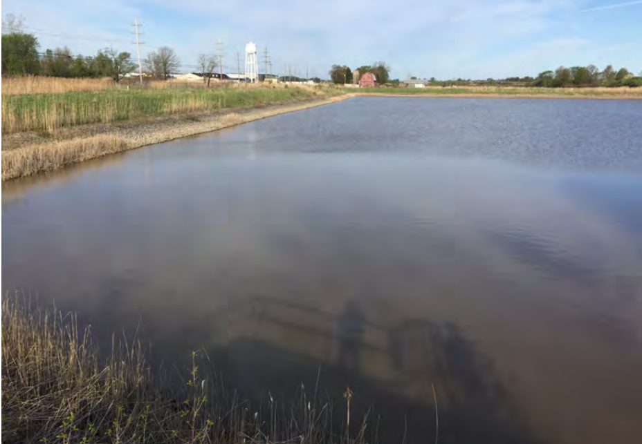
1. Storm Water Detention Basin (SWDB), S & W Sides. Slopes are Protected with Stone. No Visible Slope Erosion on All Sides. Same for N & E Sides.
