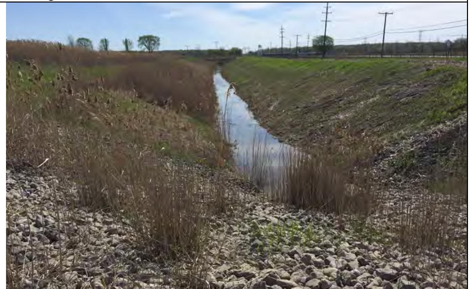
28. Perimeter Ditch Along South Side Looking East.
