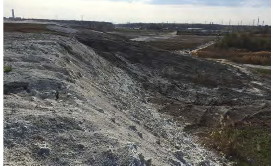
32. Temporary Slope of CCR Placement Southwestern Side.
