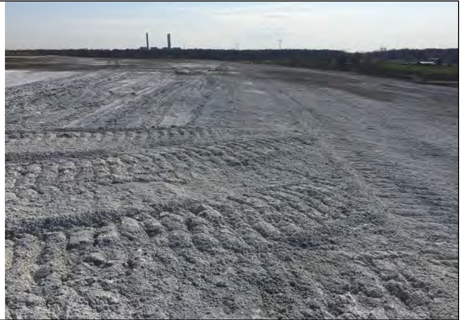
38. Another View of Graded Landfill CCR Sloped Surface.
