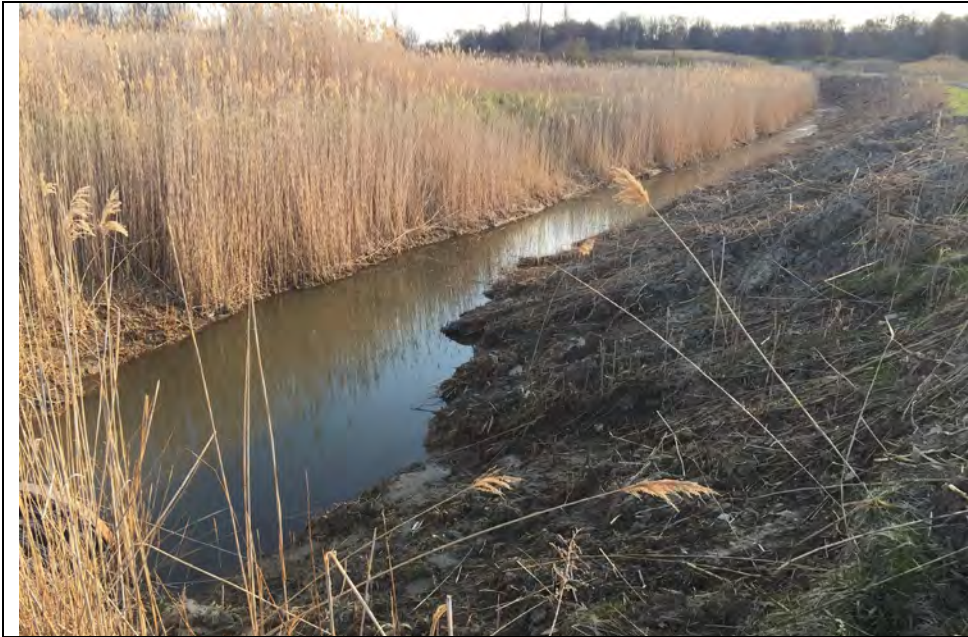
5. Ditch Maintenance Along One Side where Access from Road Easiest.
