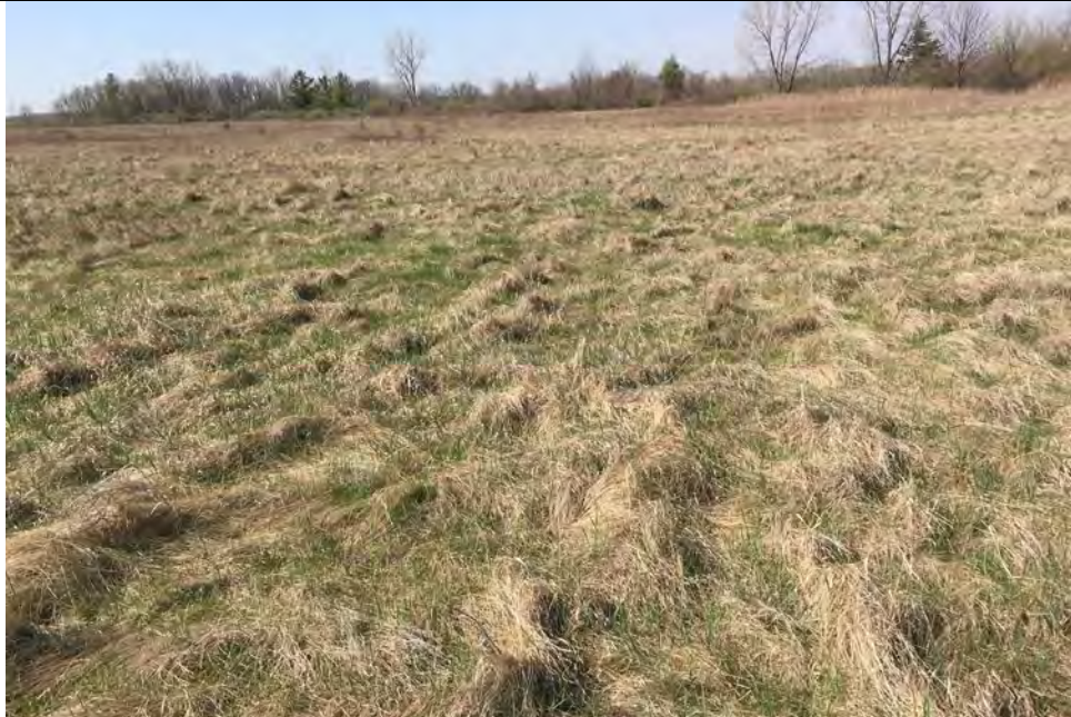
53. Typical Top of Landfill in Historically Closed Areas. Well Vegetated with Occasional Brush Growth, as Shown in Distance.
