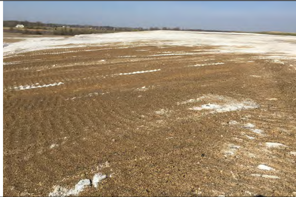
37. Another View of Graded Landfill CCR Sloped Surface. Area G2.
