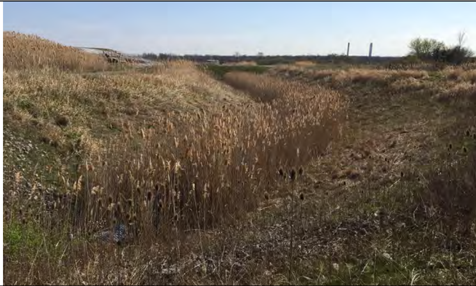
43. Perimeter Ditch Looking East.
