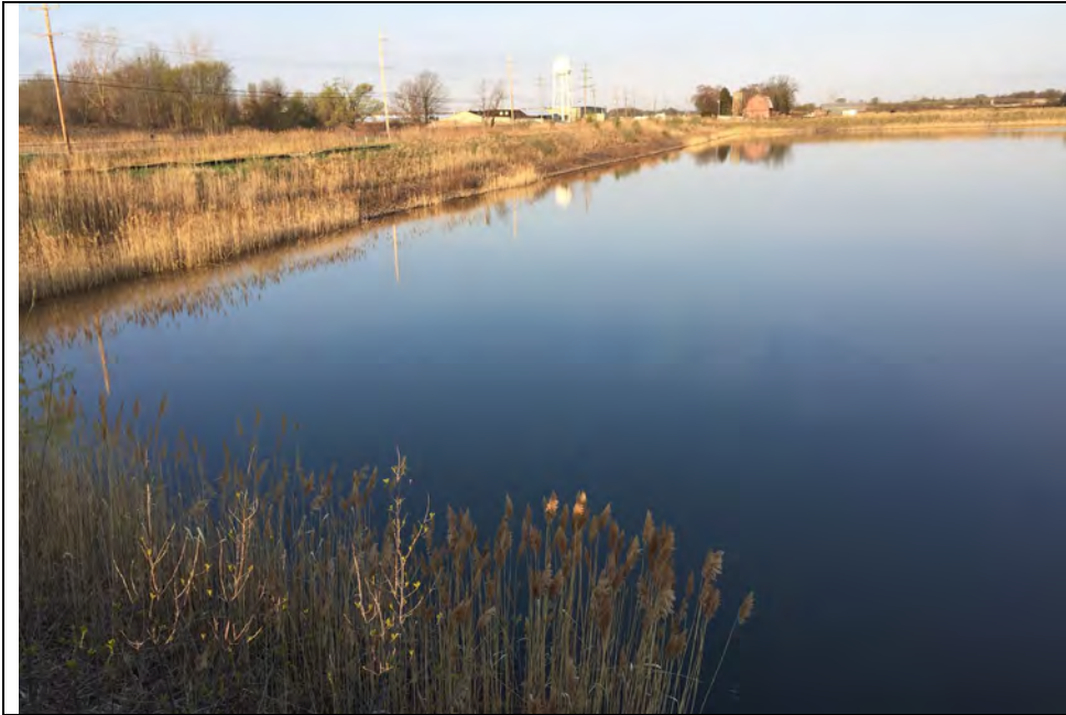
1. Storm Water Detention Basin (SDB), S & W Sides. Slopes are Protected with Stone. No Visible Slope Erosion on All Sides. Same for N & E Sides.
