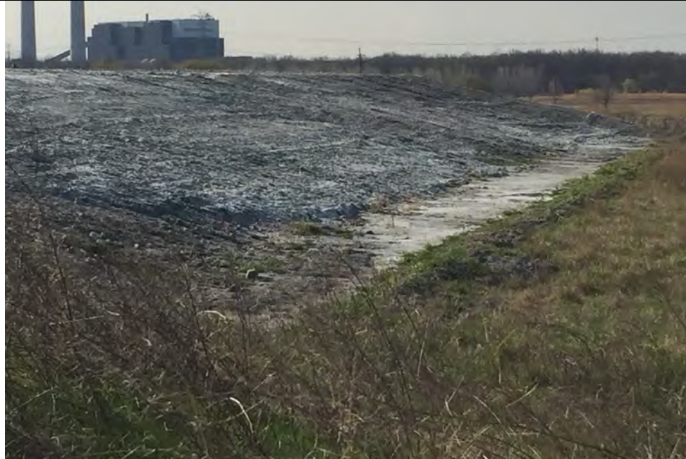
29. View of South Side of Active Disposal Area Slopes. Photo Taken from Outside of Active G2 Area Along the West Side Existing Berms.
