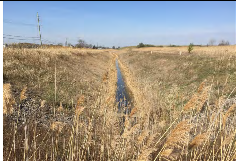
42. Perimeter Ditch Looking West Along South Side Near Puttygut Road.
