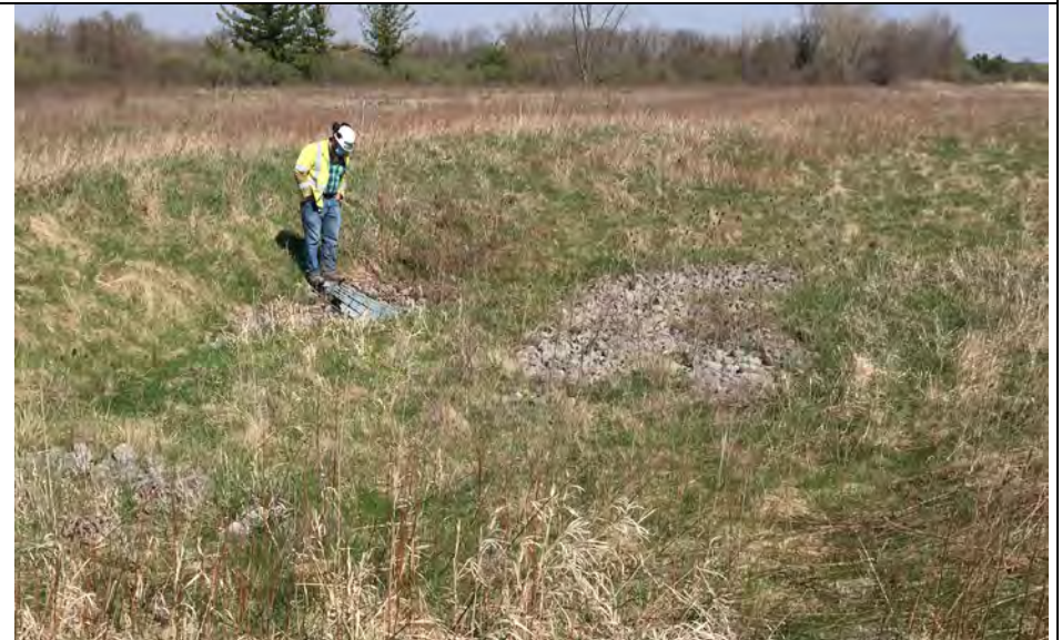
52. Inlet Side of Downslope Drainpipe with Small Riprap Grading to Prevent Gully Erosion.
