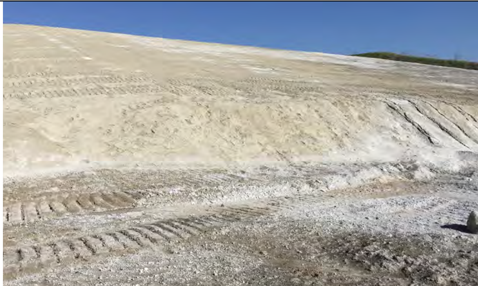
35. Active CCR Slope with Grading InProgress. Area G2.
