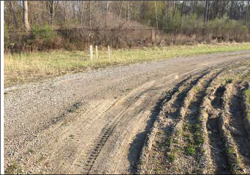
21. Perimeter Road and GW Monitoring Well 16-06. Well Protected and Locked. Unusual Rutting from Maintenance Equipment Used as Part of Ditch Cleaning.
