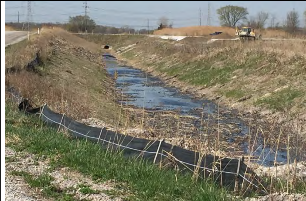
41. Internal Drainage Ditch Located South of Active Area G2
