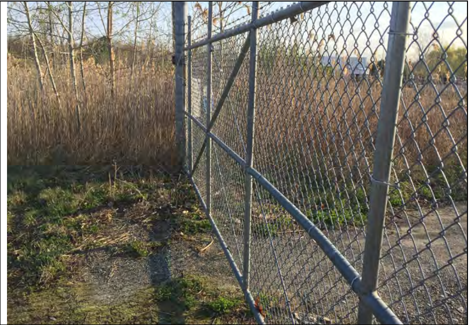
10. Side View of Locked Gate with Signage. All Gates observed had Signage and were Locked.
