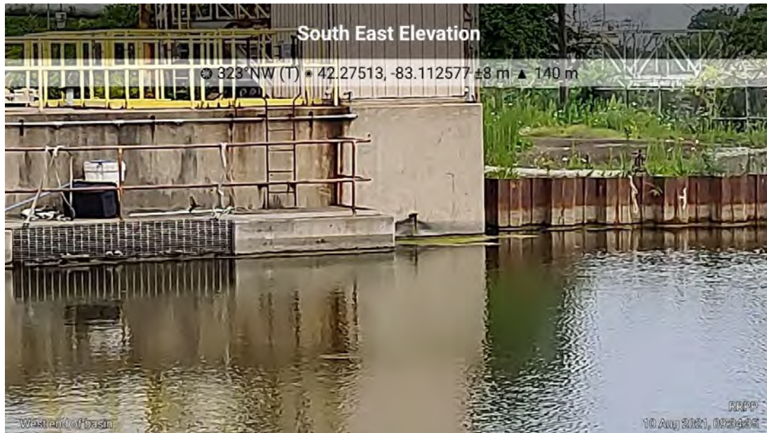
Photograph 8: Pump House Sump Pump Looking West from North Side of Basin
