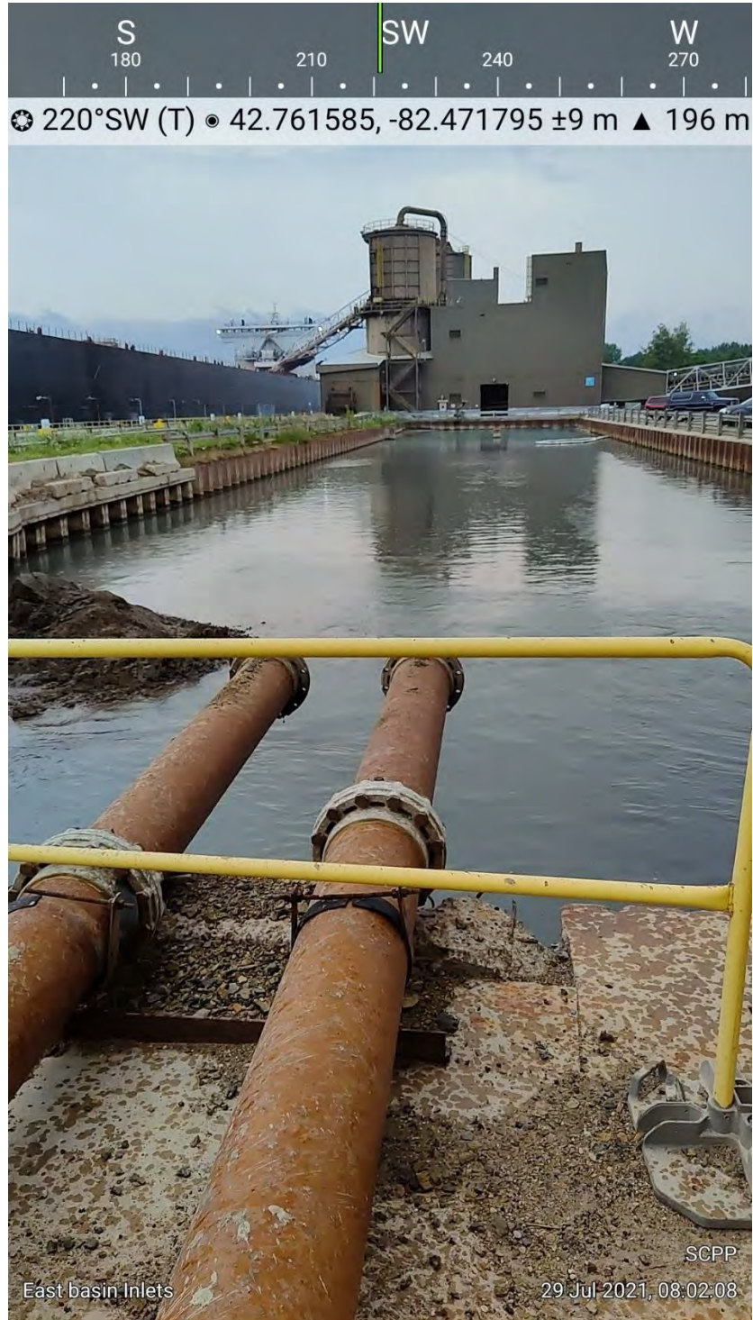
Photograph 3: East Basin Looking South from North End
