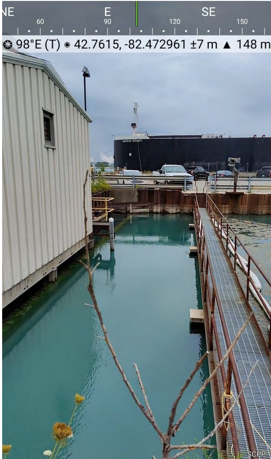
Photograph 7: West Basin Weir Looking East from Northwest Corner of West Basin
