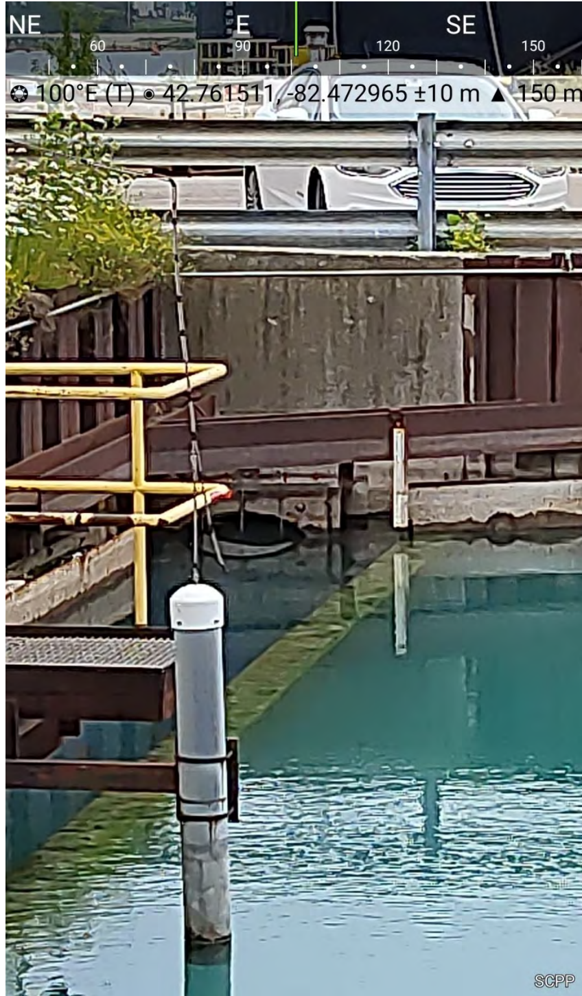
Photograph 8: West Basin Outlet Looking East from Northwest Corner of West Basin
